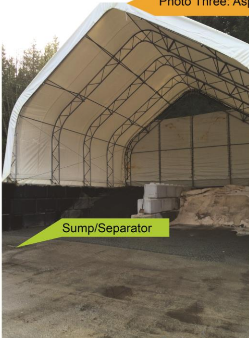
Photo Three: Asphalt pad and sump
