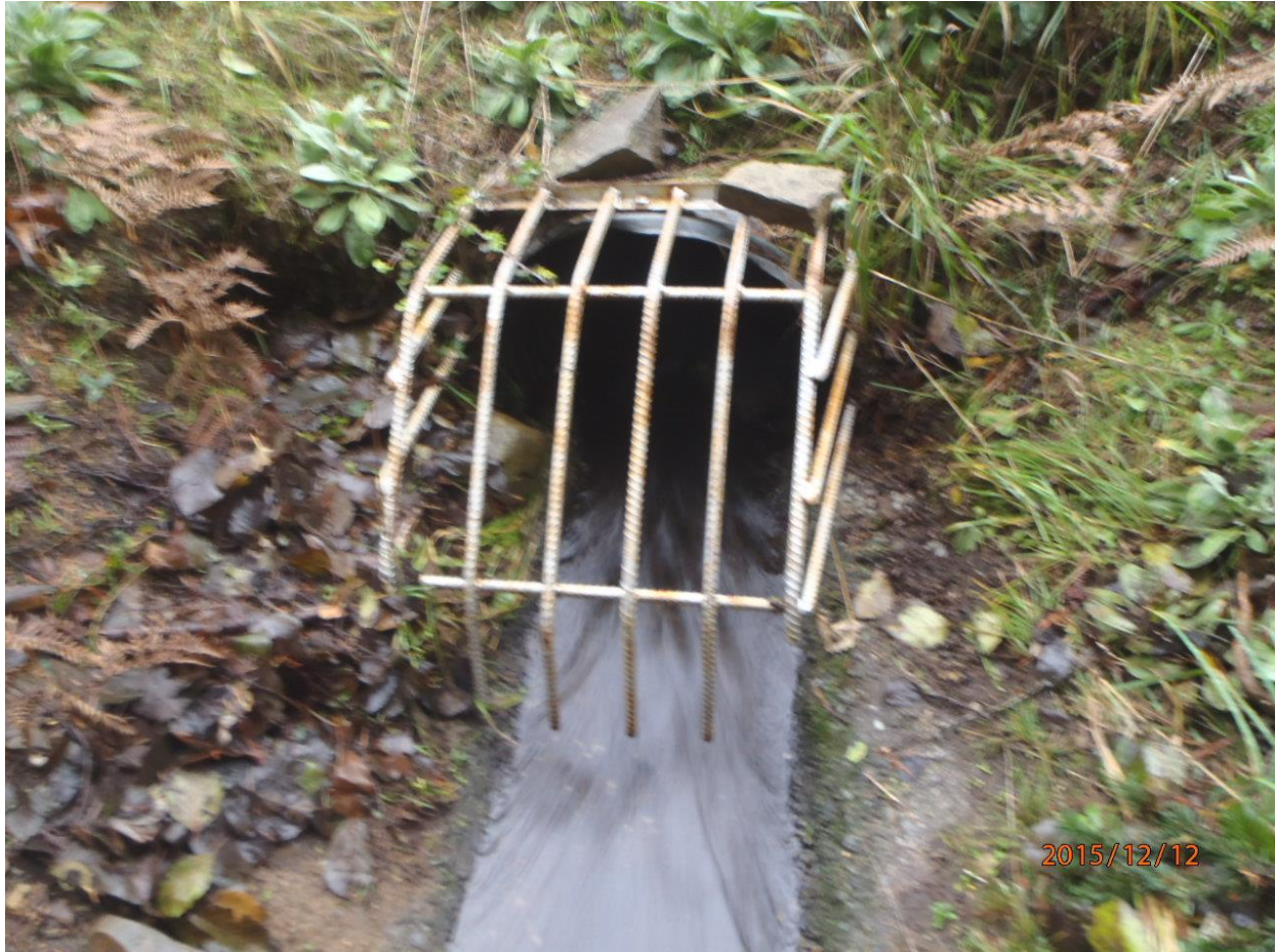
Photo 2. The inlet culvert under Galleon Way
