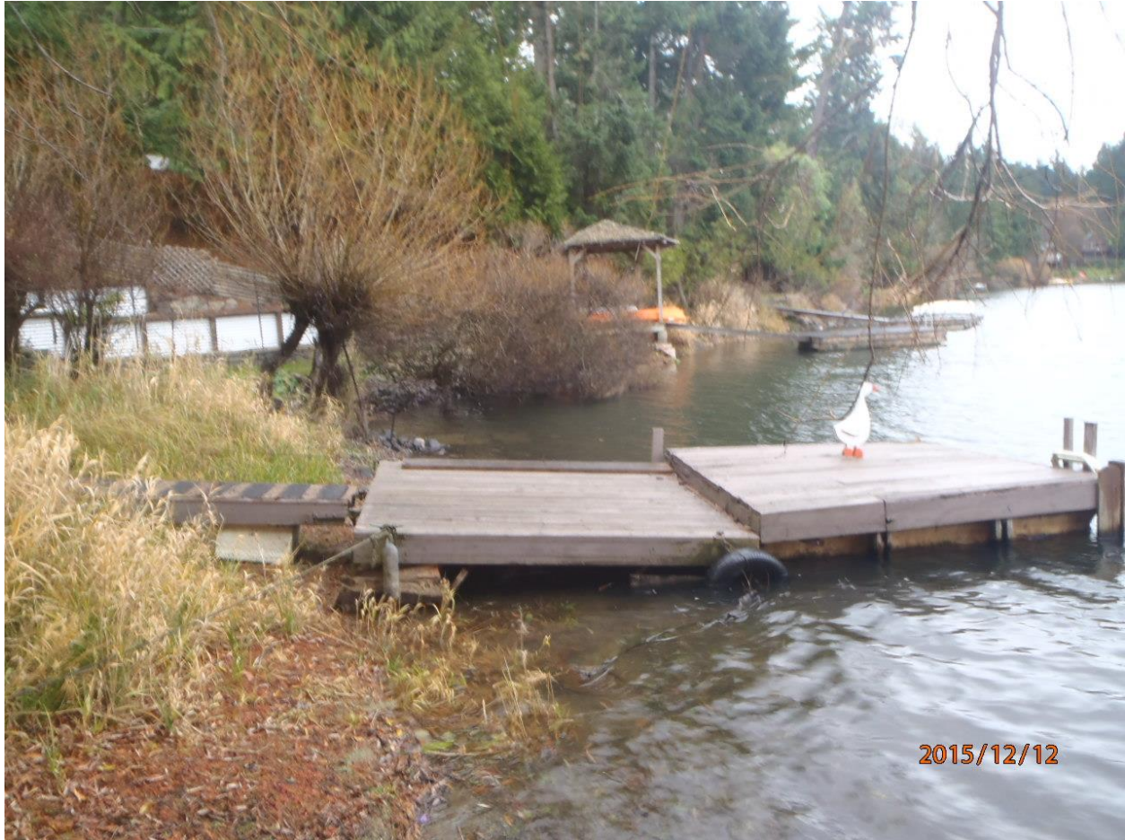
Photo 3. Buck Lake shoreline is in stable condition
