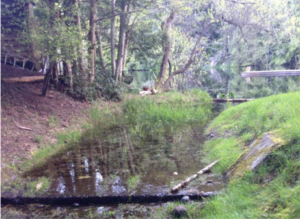
Photograph 3. The outlet of Magic Lake—cement weir sets the high water level
