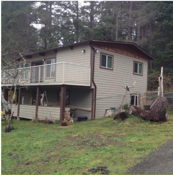
Photo One: Subject Accessory Building from South
