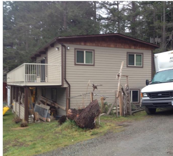
Photo Two: Subject Accessory Building from East
