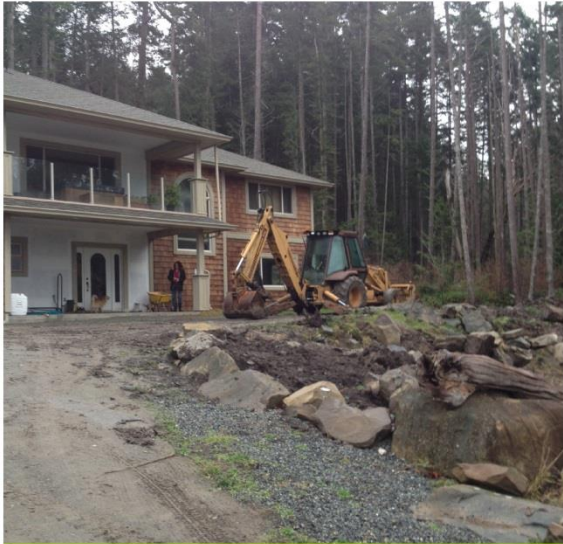
Photo Three: Main Dwelling on Property
