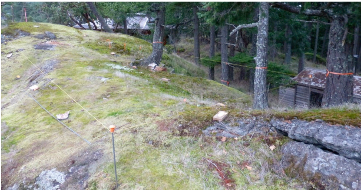
Figure 13. The cottage's footprint at the top of ridge. Trees marked with flagging tape are to be removed.
