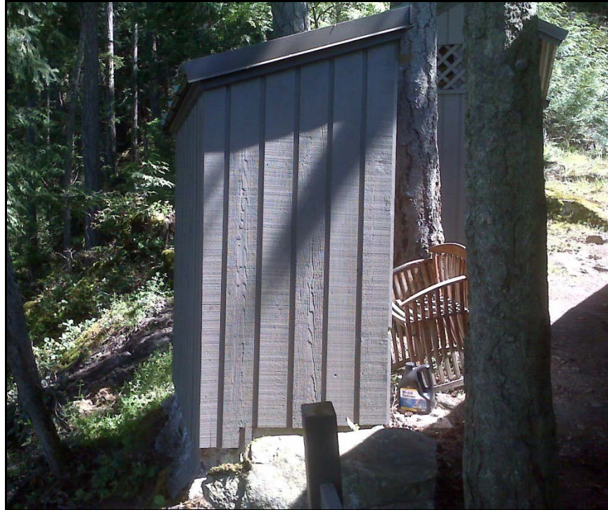
Photograph 3: The Shed Containing a Propane Tank (Shed in Distance complies with setback)
