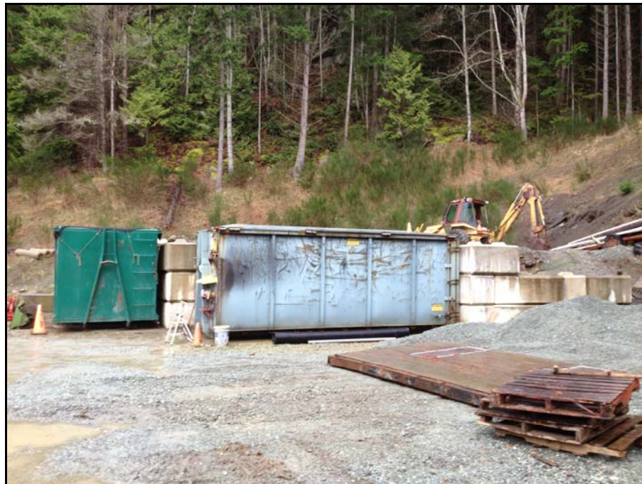
Photograph 1: Upper Level - Waste Storage and Recycling Location
