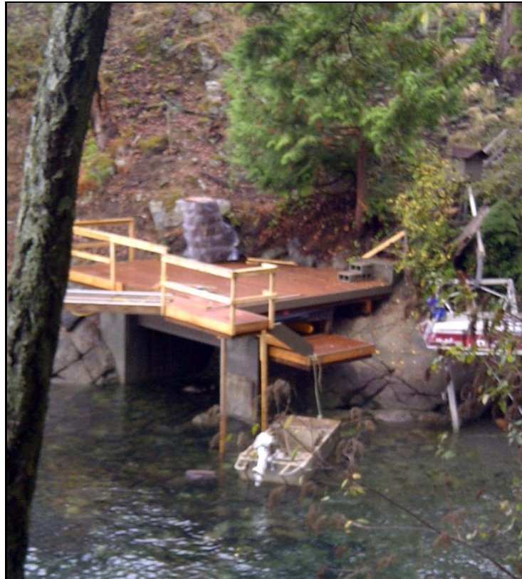
Photograph 11: Foreshore Deck, straddles the Natural Boundary
