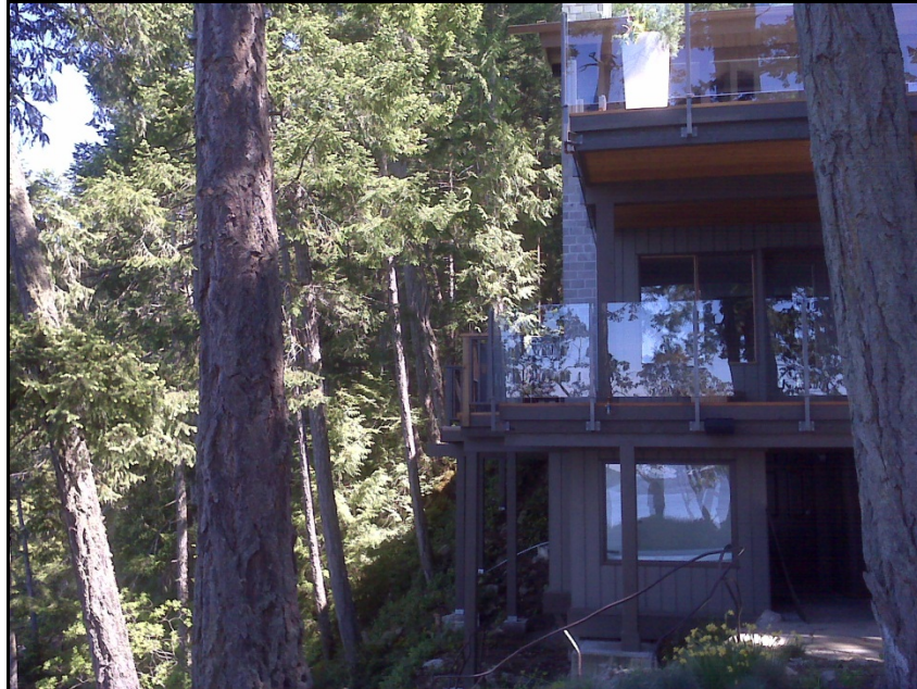
Photograph 1: Looking West along Northern Side of Dwelling
