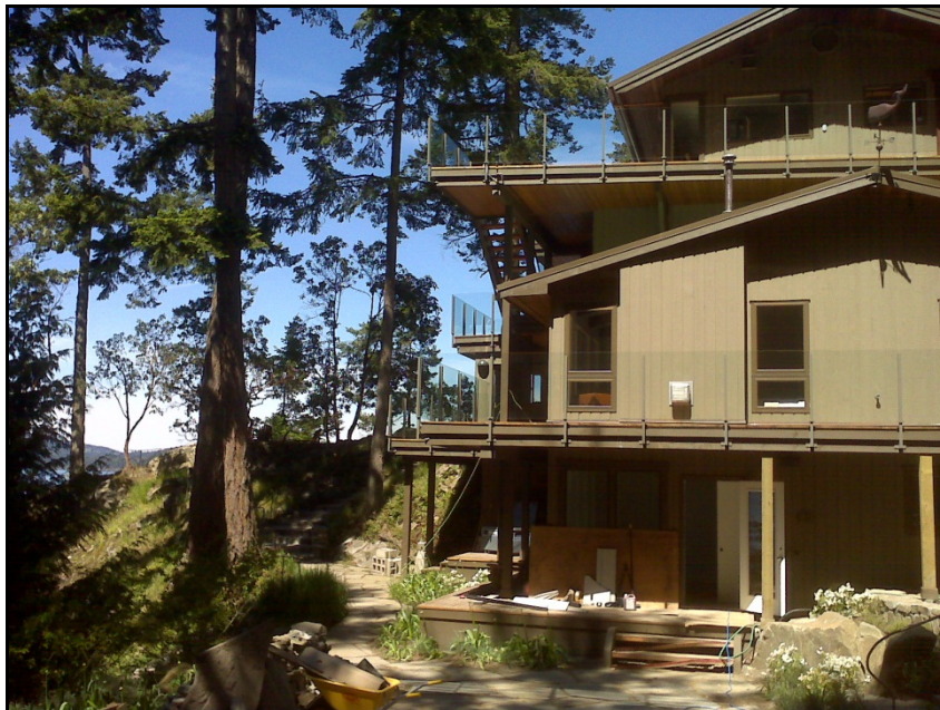
Photograph 2: Looking North along Western Side of Dwelling
