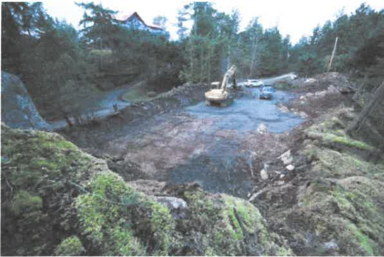
Figure 1 Looking Southwest from on the large ridge east of proposed building. Beyond is the north side of BnB to the south
