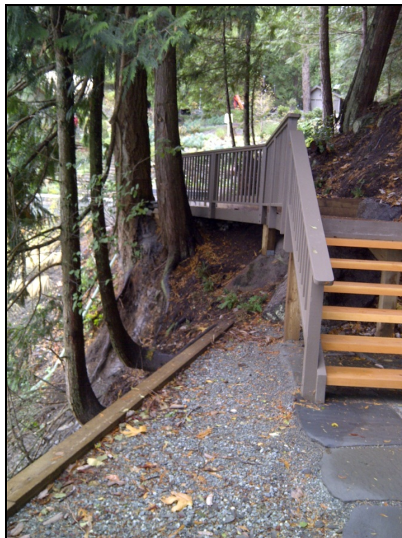
Photograph 8: Wooden Walkway, Looking Westward toward the Main Patio
