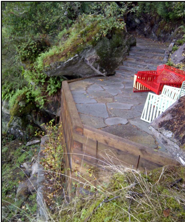
Photograph 10: South Patio and Retaining Wall
