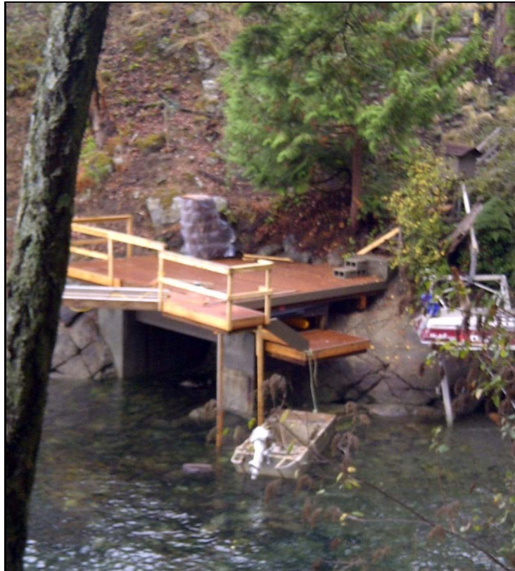
Photograph 11: Foreshore Deck, straddles the Natural Boundary
