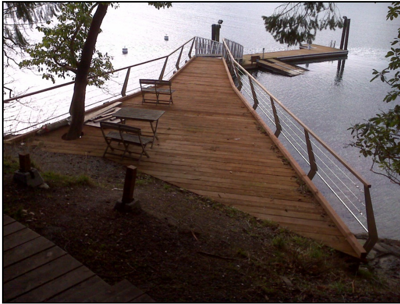
Photograph 1: Upland End of Walkway
