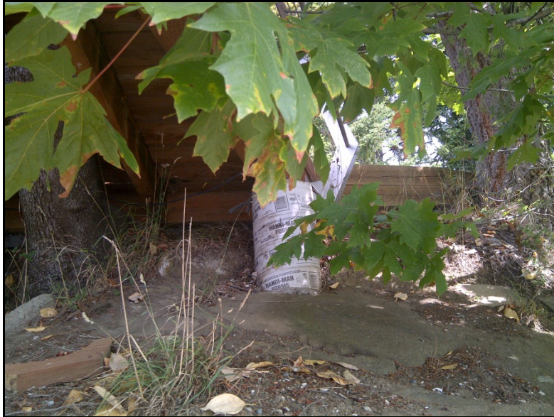
Photograph 3: Underside of Walkway, Arbutus Tree on Left and End of Gravel Pathway on Right
