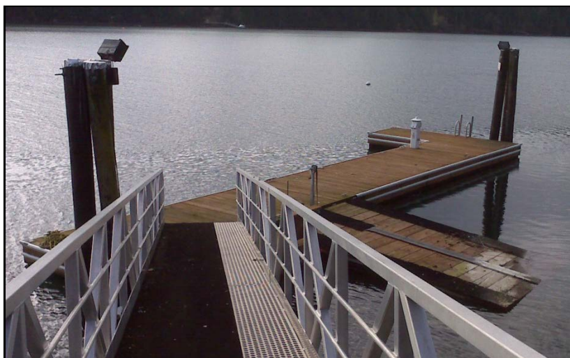
Photograph 3: Float With Boat Ramp to be Removed, and Seaward Side Projection to be Reduced in Size
