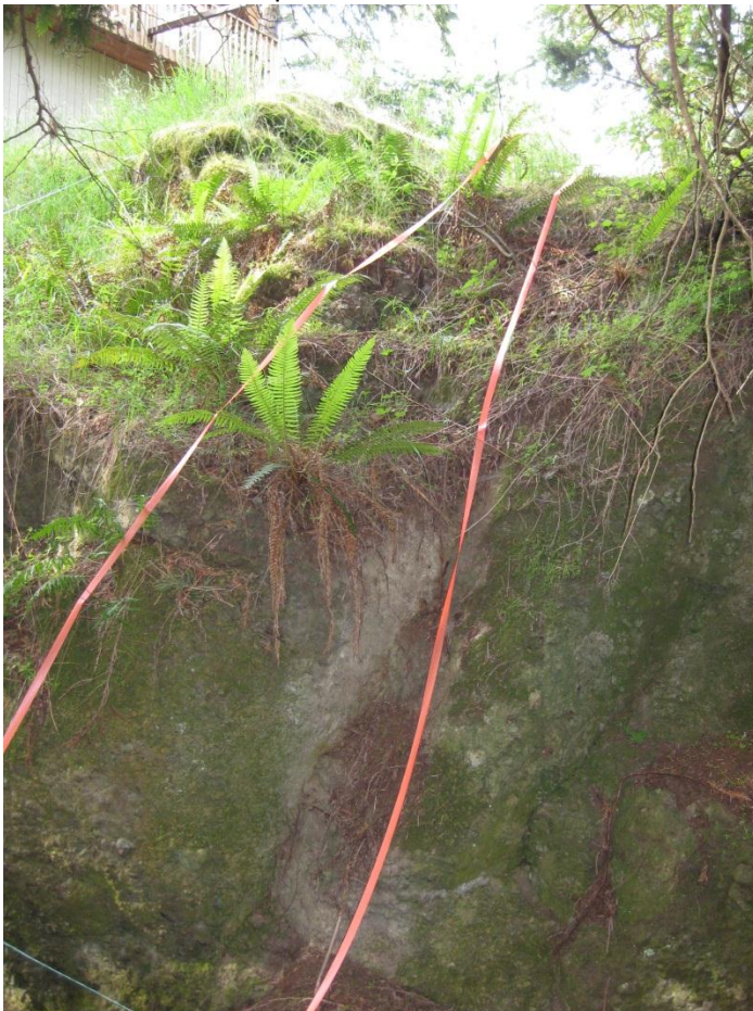
Photo 8 Rock outcrop in area of stair construction
