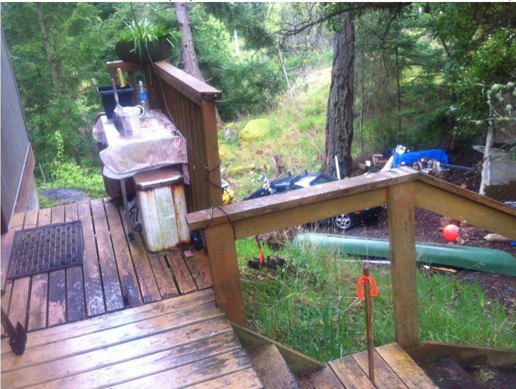
Photo 2 Non-sensitive area proposed for entrance/mudroom and deck construction (west side)
