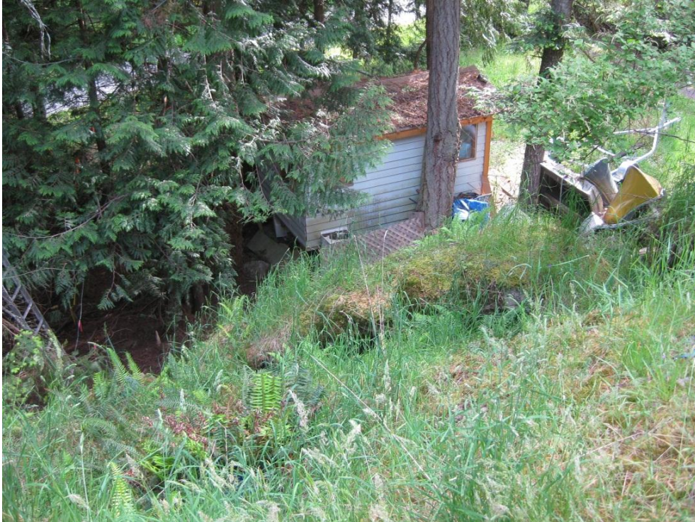
Photo 7 Area proposed for stair construction from deck to garage (see rock outcrop detail below in Photo 8)
