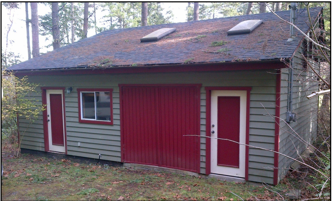
Picture 2: Accessory Building Near Entrance (Variance granted 1993)
