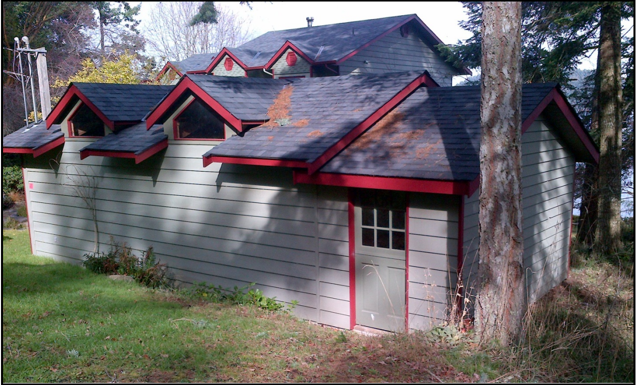
Picture 1: Outbuilding Requiring Building Permit and Setback Variance
