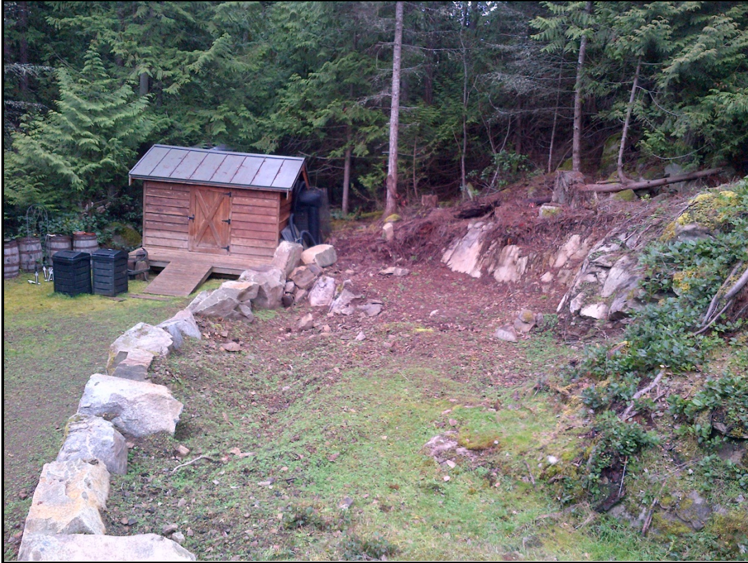
Photograph 1: Location for proposed sauna and existing accessory building.
