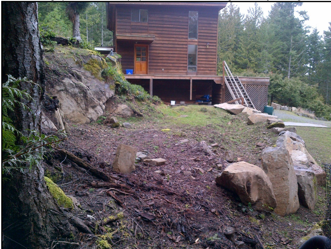
Photograph 2: Sauna site location and dwelling
