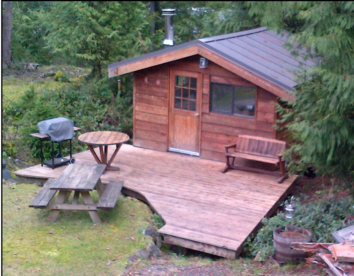
Photograph 3: Existing accessory building as part of variance to legalize siting
