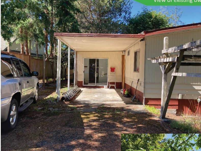
View of existing dwelling from driveway
