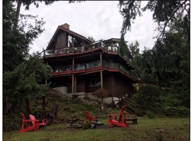
Image 8: Rear view of subject dwelling unit.
