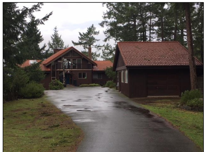
Image 6: Front view of subject property.
