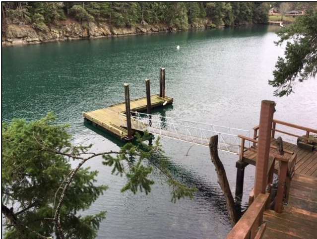
Image 9: Dock at subject property.
