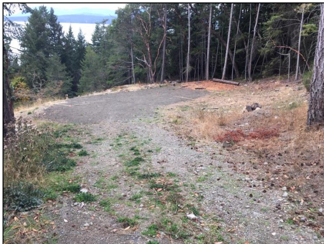
Image 4: View of cleared building site on Lot 7.
