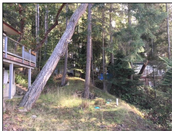
Image 6: Proximity of subject dwelling to dwelling on adjacent southern lot
