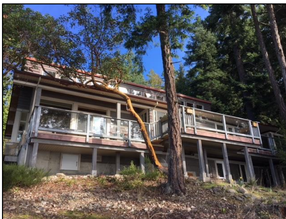
Image 4: West elevation of subject dwelling
