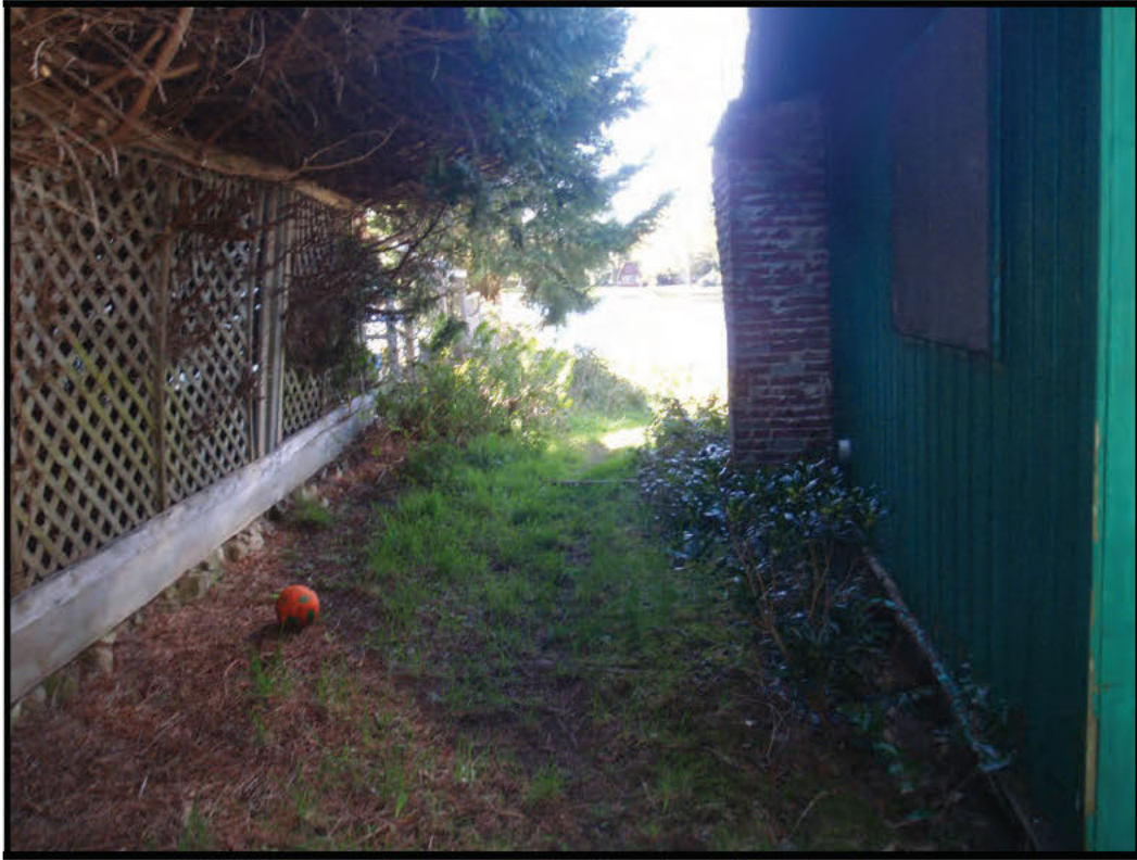
Photograph 3. View south along east side of existing house.
