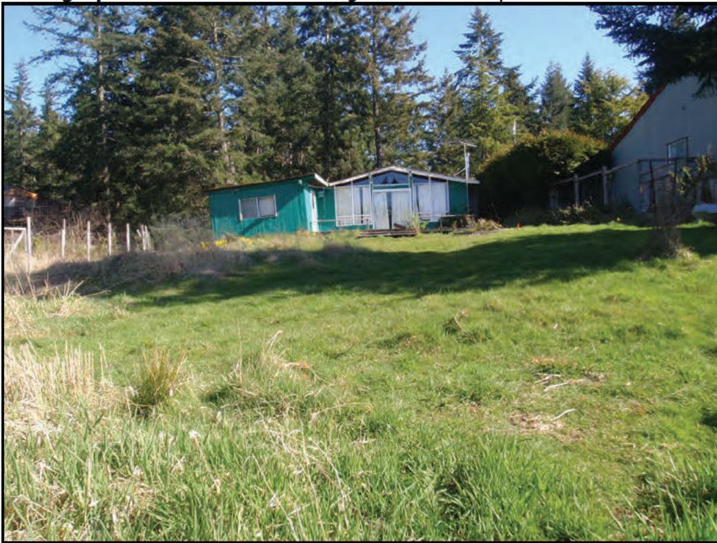
Photograph 8. View north towards house that will be replaced.
