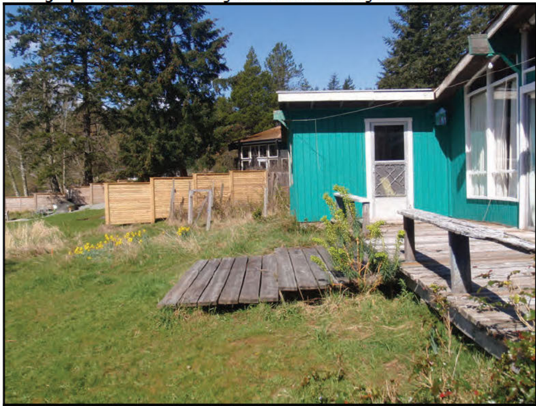
Photograph 4. View west along south side of existing house.
