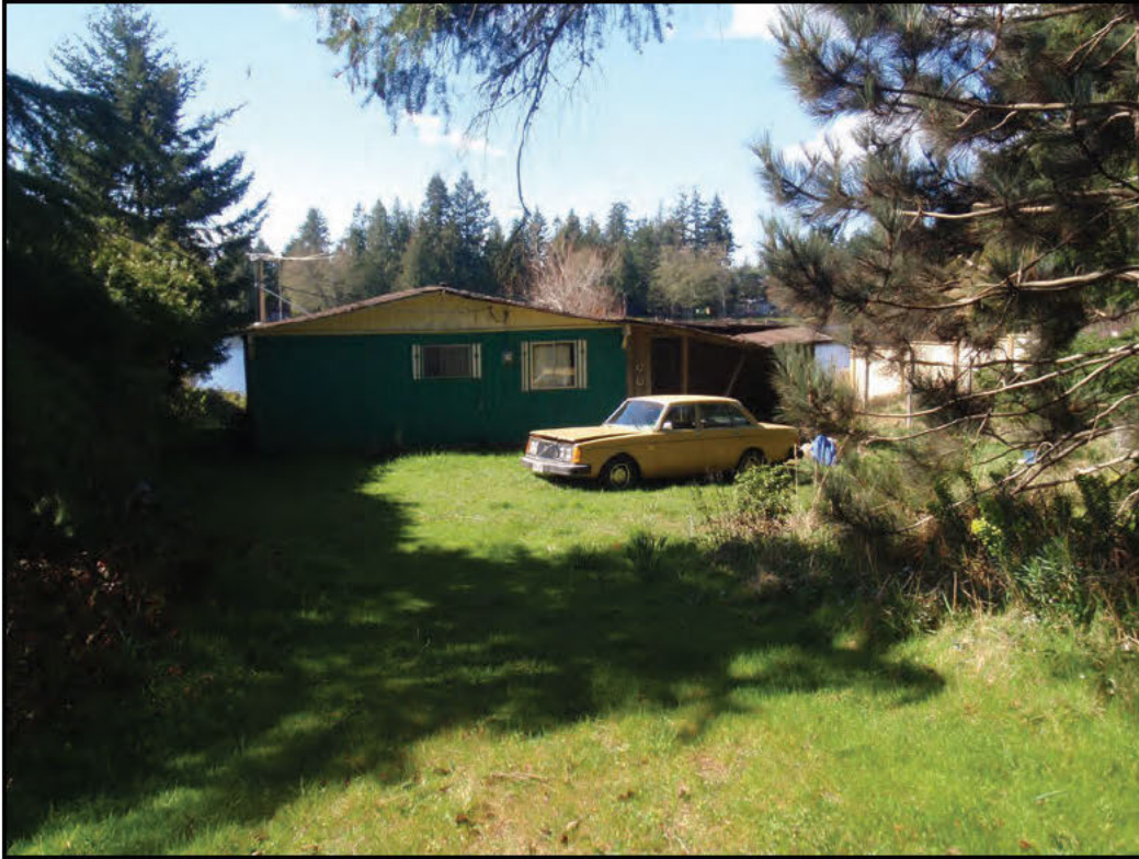
Photograph 7. View south of existing house to be replaced.
