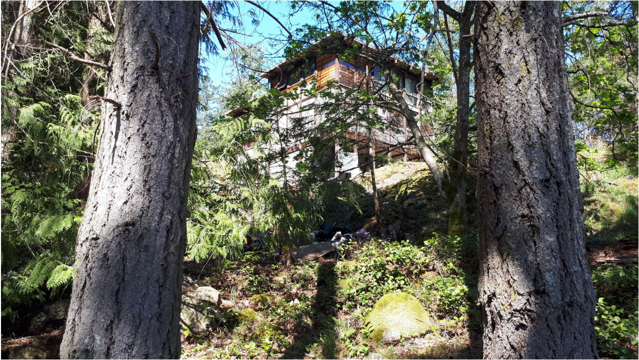
Plate 5. Northwestern side of subject property showing view of adjacent development.
