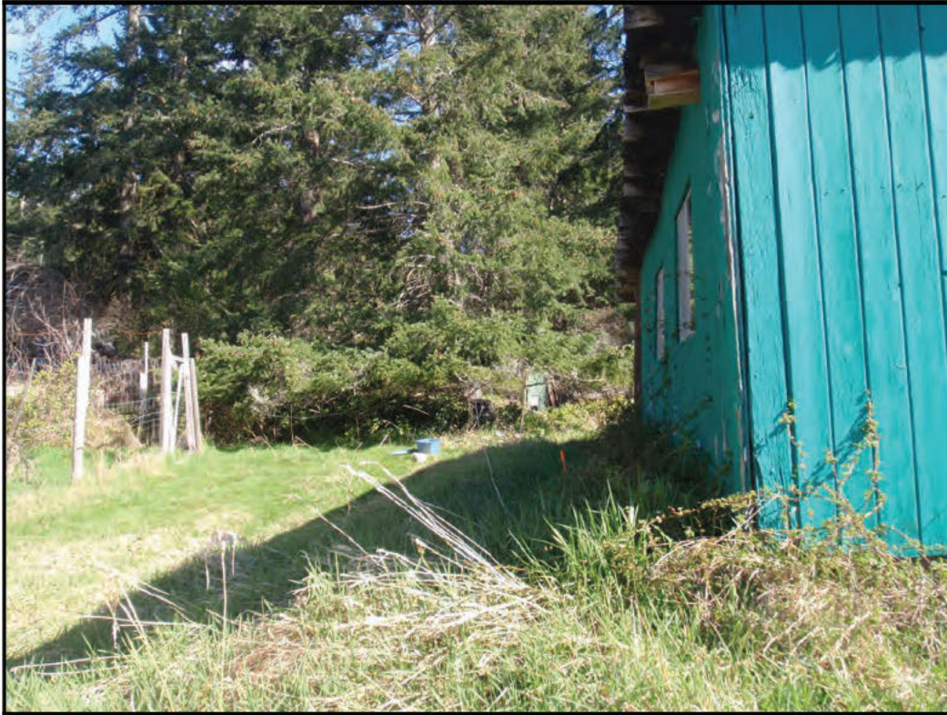
Photograph 1. North view along west side of existing house.
