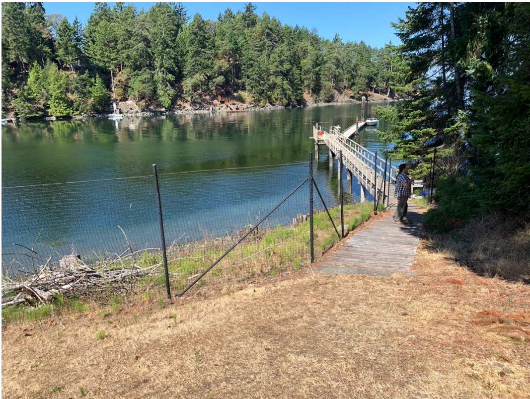
Photo 14. Existing dock and beach access.
