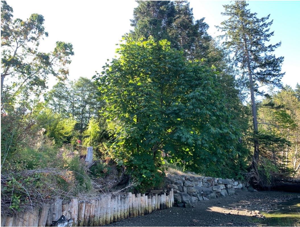
Photo 3. Looking south along the shoreline at the junction of the failing log structure and stacked boulder wall on the adjacent property. Temporary beach access by heavy equipment proposed for this section.
