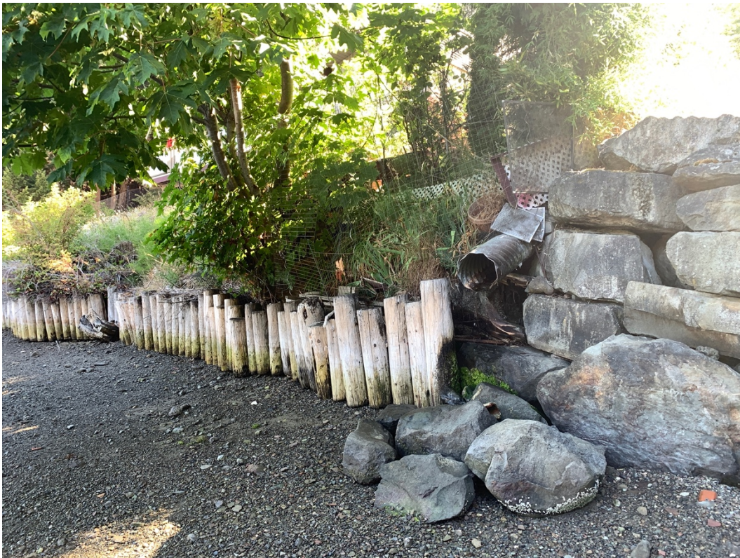
Photo 4. South end of the site: the proposed wall will be integrated with the existing stacked boulder wall to the south, incorporate the stormdrain outfall, and support the existing bigleaf maple. Retention of the maple will require temporary beach access for the heavy equipment.
