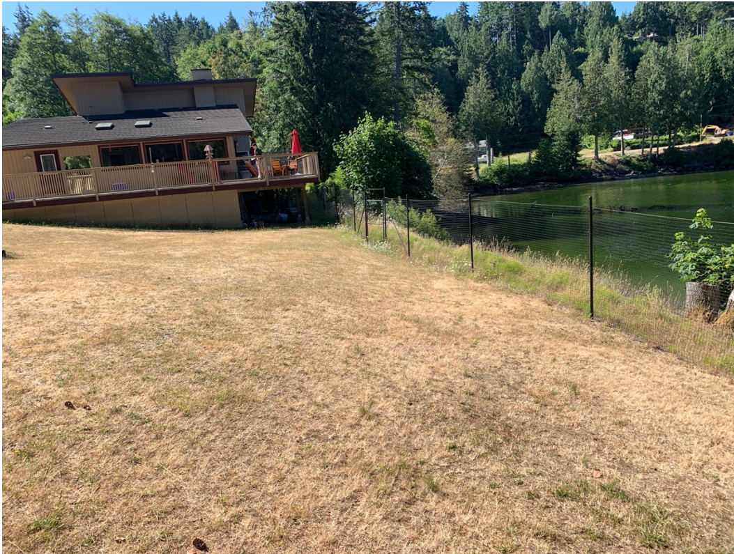
Photo 15. Looking south along the top of bank, work will be conducted from the top of the slope.
