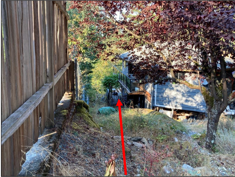
VIEW FROM SEXTANT ROAD (LOCATION OF DECK EXTENSION NOTED BY ARROW)
