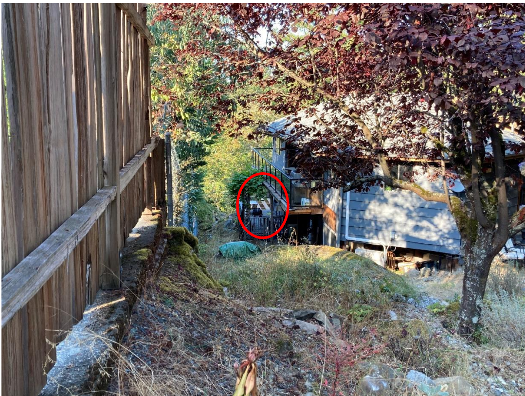
Picture One – View from Sextant Road looking west towards subject dwelling (area in red notes area of new deck extension)
