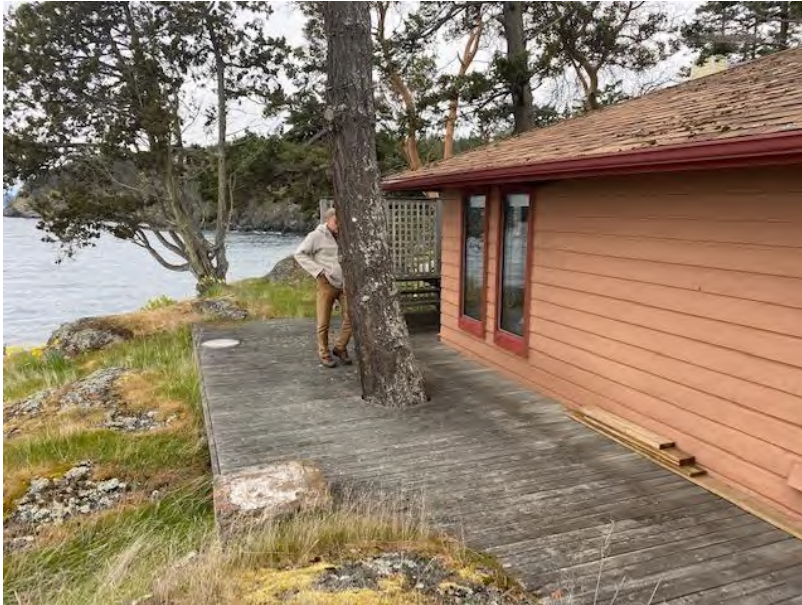
MARINE SIDE OF EXISTING DWELLING
