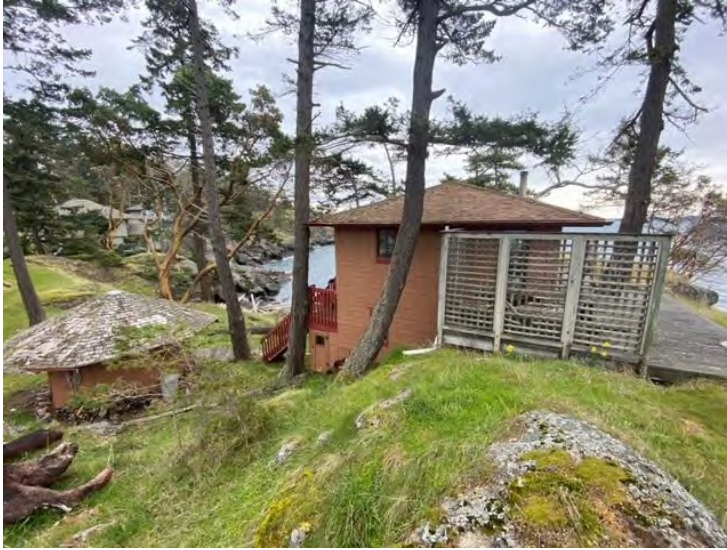
SIDE OF HOUSE AND EXISTING SHED
