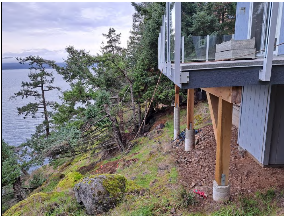
2.3.2 Deck attached to dwelling, looking north-west
