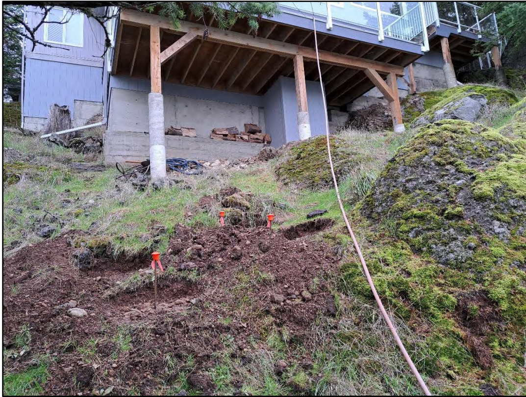
2.3.3 Stairway foundation location and deck, looking north-east
