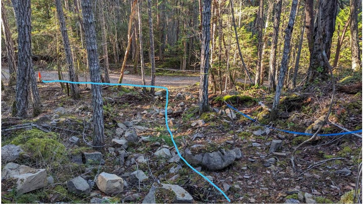
Photo 10: Shows the route of the buried water line (bright blue) with the wellhead located in the top left of the photo with an orange cone on top. The blue flagging on the right of the photo roughly indicates the northern edge of the proposed house.
