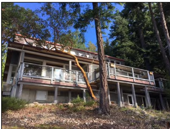
Image 4: West elevation of subject dwelling
