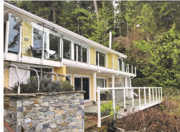
Dwelling's northwest elevation
