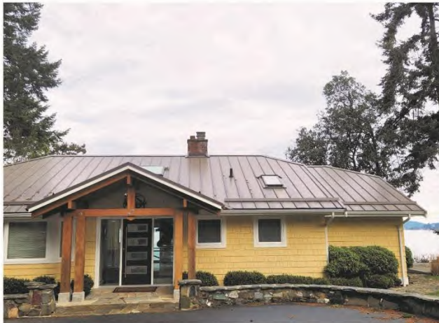
Dwelling front entrance (southeast elevation)
