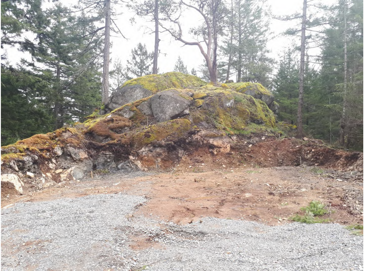
Figure 2. Area of clearing looking east along the western edge of the Woodland DPA at 5909 Pirates Road.
