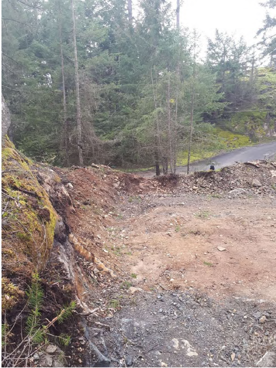
Figure 3. View looking North where slope levelling is needed to prevent erosion of dug out slope.
