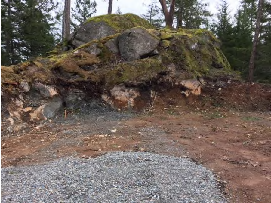
LOOKING WEST FROM EXCAVATION
