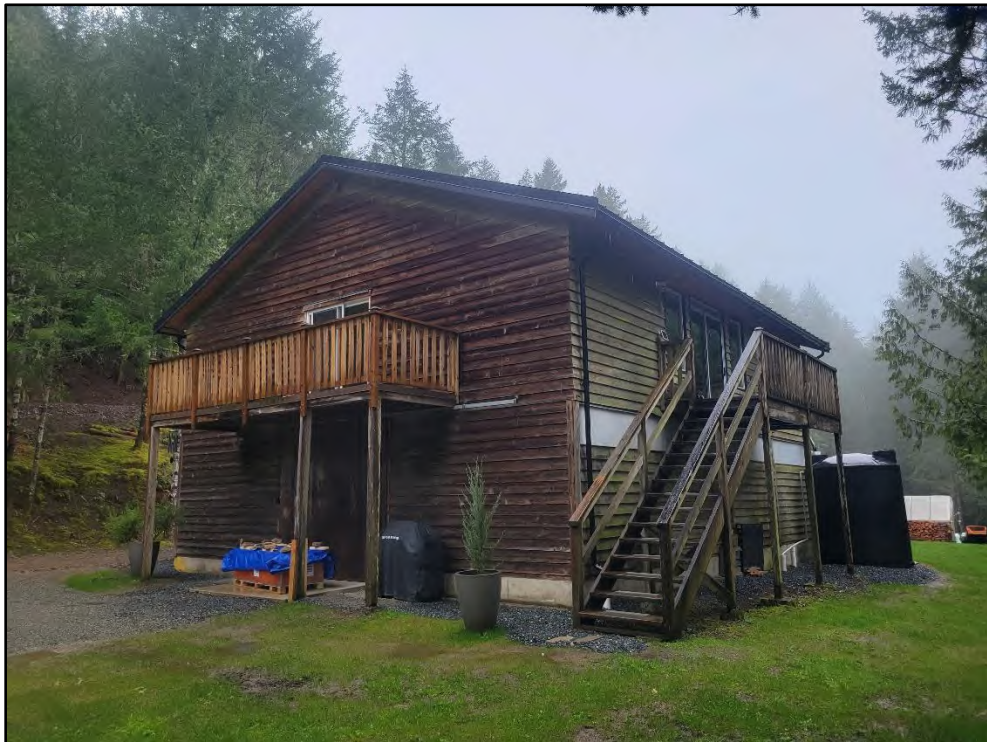
EXISTING BARN, LOOKING WEST
