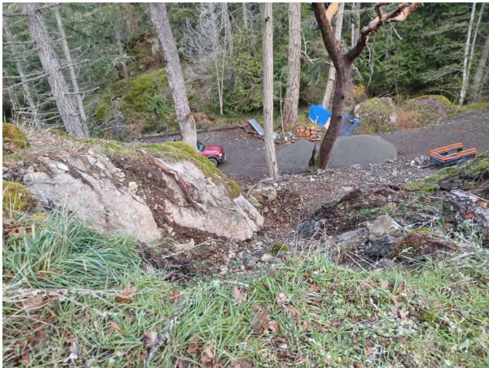
Plate 6. Newly constructed driveway and adjacent utilities corridor along the boundary of the Herbaceous Ecosystem DPA at 6915 Pirates Road, Pender Island, BC.
