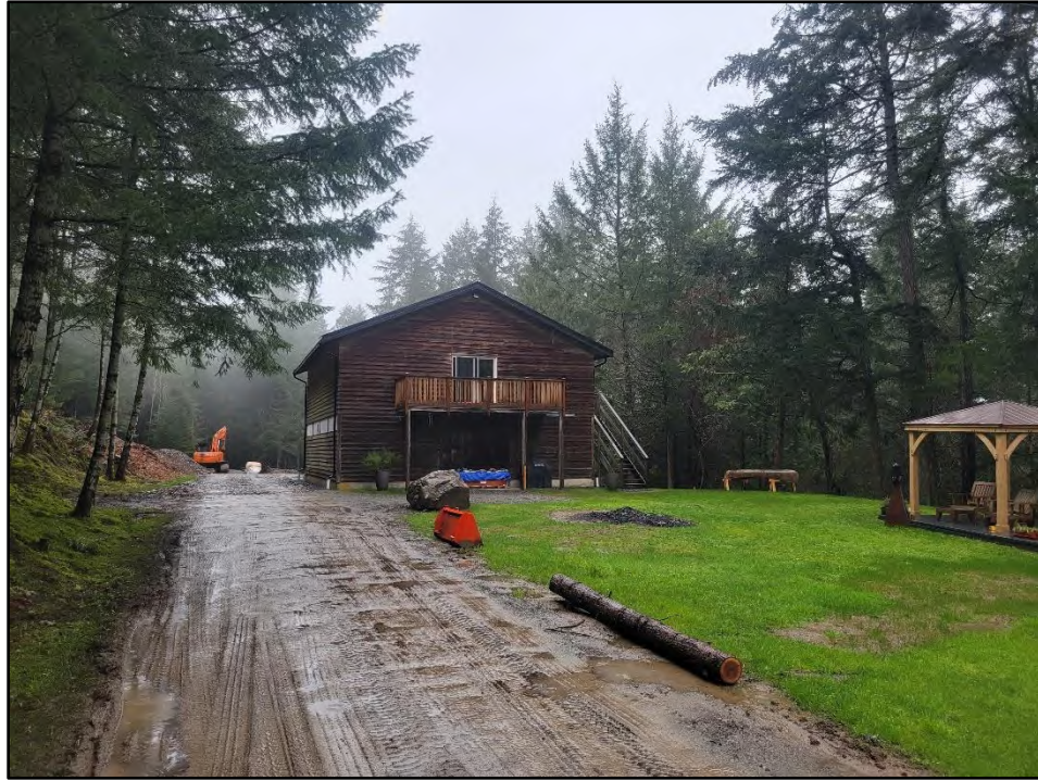
EXISTING BARN, LOOKING NORTH-WEST
