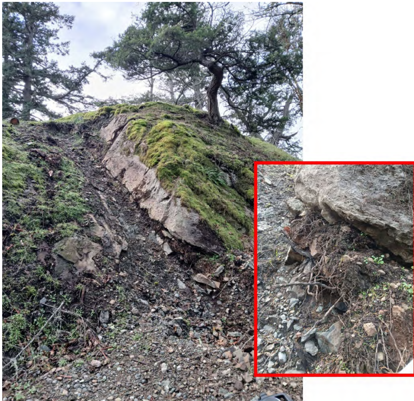
Plate 3. Disturbance to the Herbaceous Ecosystem DPA with exposed tree and shrub roots (inset), causing erosion risk following construction of utilities access corridor at 6915 Pirates Road, Pender Island, BC.
