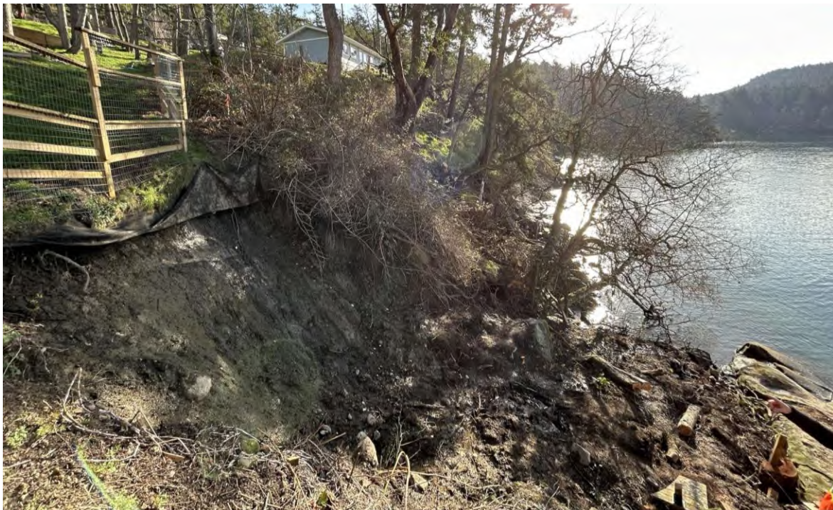
Photo 3: Looking SE at landslide. Note soil and debris in runout path, with sandstone bedrock on beach.
