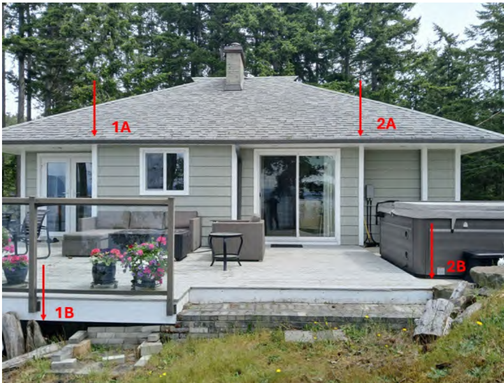
Plate 2. Uncovered back deck with locations of anchoring points at current roof (1A, 1B), and anchoring points at edge of current deck (2A, 2B) at 2705 Yawl Lane, Pender Island, BC
