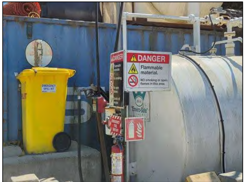
Photo 5: Diesel storage in double walled container with full sized spill kit next to it.
