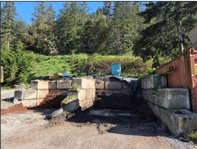
Photo 3: Soils are contained in lock block bins.
