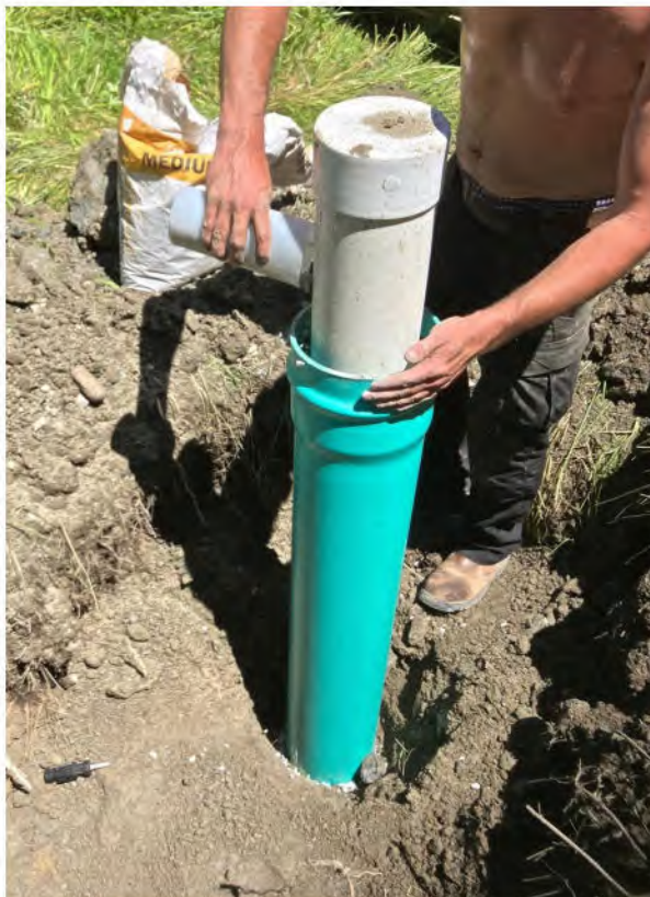
Photo 7. Pouring bentonite pellets between 6 inch diameter well casing and temporary 8 inch diameter surface casing, June 30, 2025.
