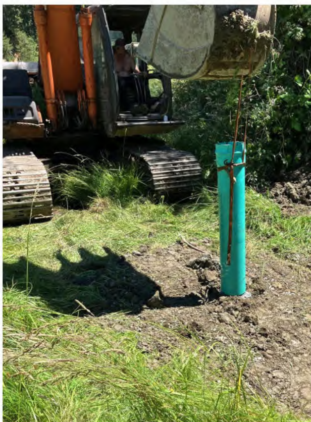
Photo 8. Pulling out 8 inch temporary surface casing, June 30, 2025.
