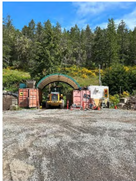
Figure 2: Site Photo Looking North
