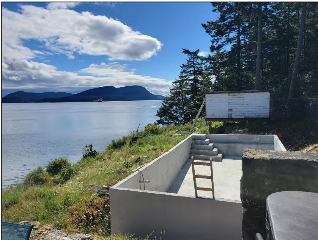
POOL CONSTRUCTION LOOKING SOUTH (2026)
