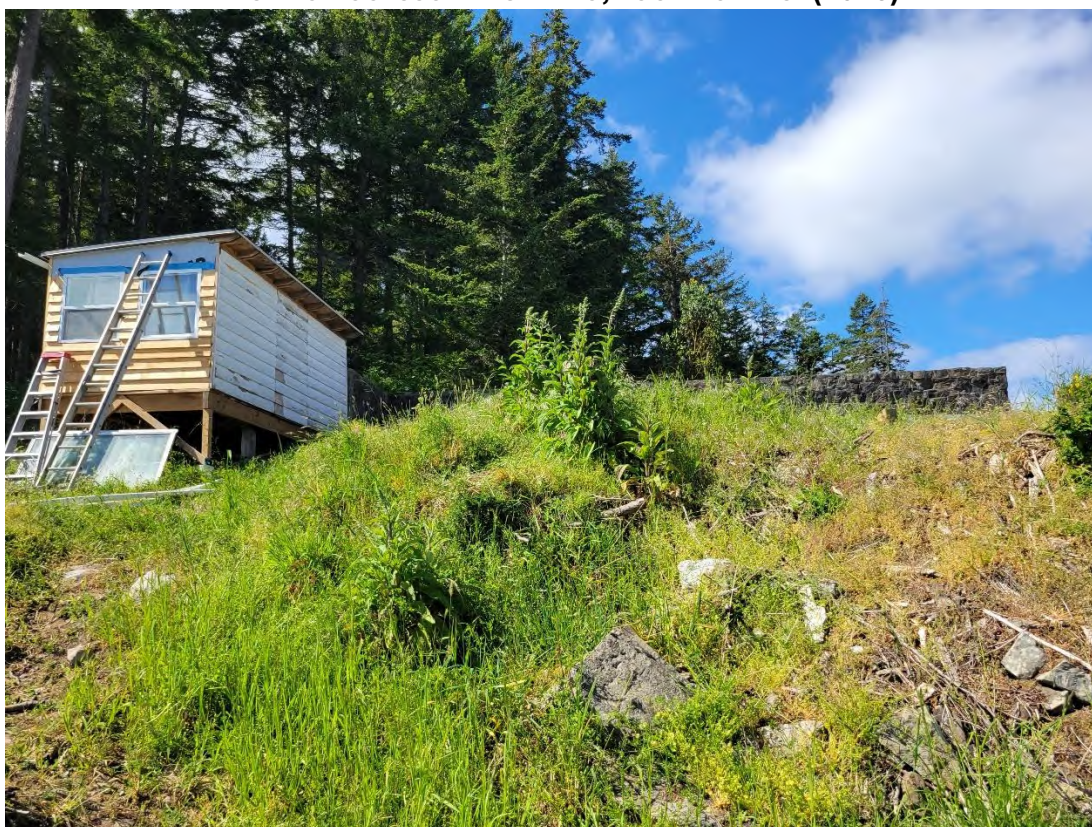
EXISTING ACCESSORY BUILDING, LOOKING WEST FROM SHORELINE BANK (2026)
