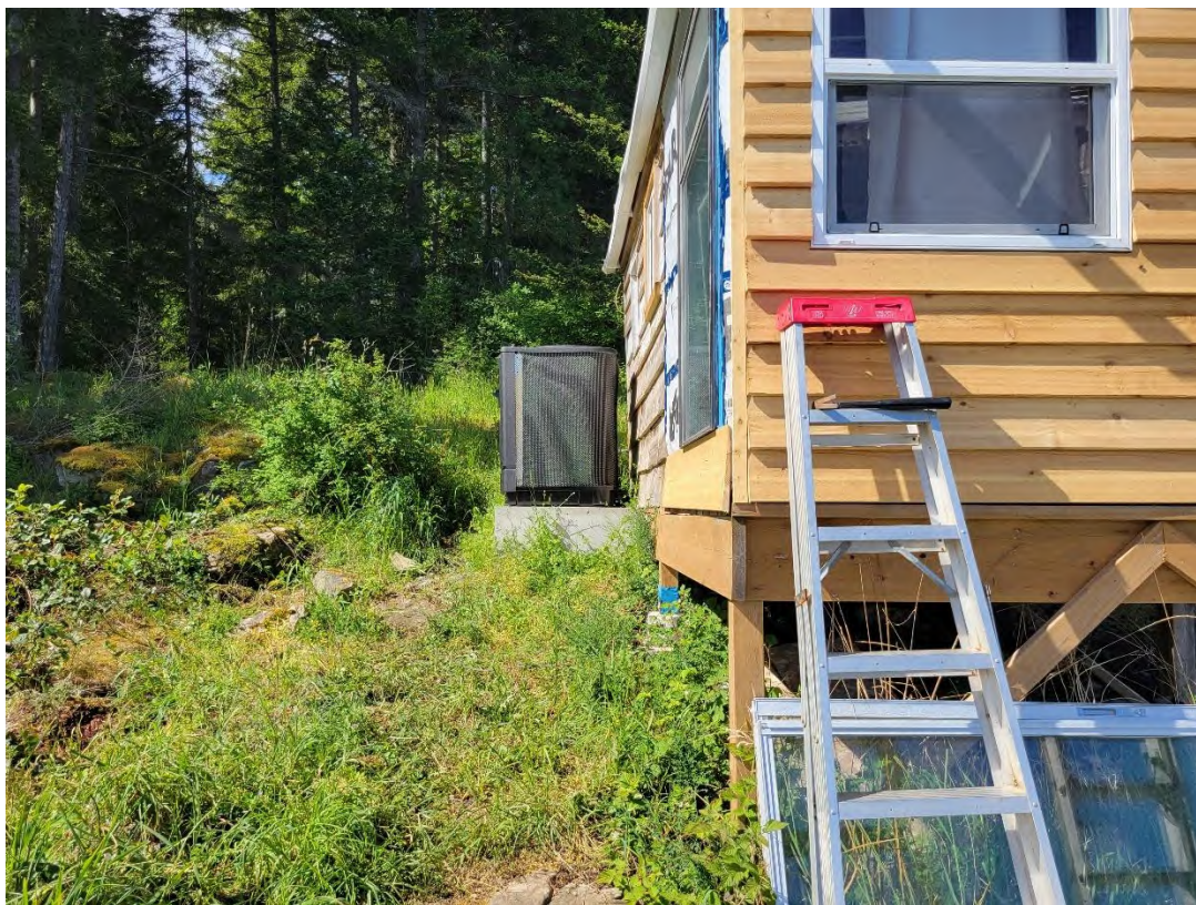
EXISTING ACCESSORY BUILDING, LOOKING WEST (2026)
