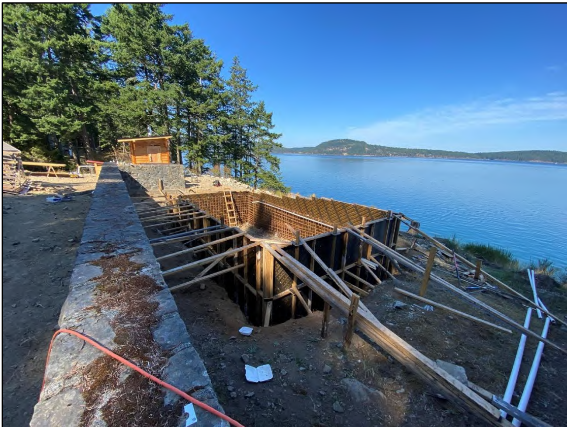
POOL LOCATION, LOOKING NORTH-EAST (2025)
