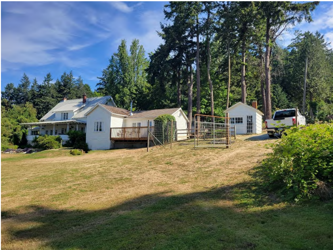
BUILDING SITE, LOOKING NORTH TOWARDS OTHER COTTAGES
