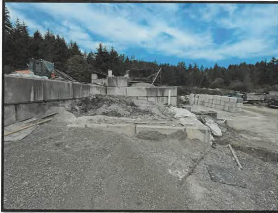
Photo 5: Solids storage area
