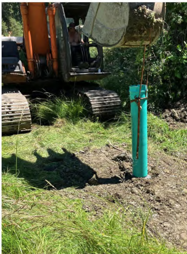
Photo 8. Pulling out 8 inch temporary surface casing, June 30, 2025.
