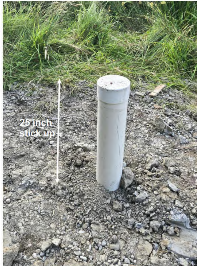
Photo 9. Completed 6 inch diameter monitoring well, June 30, 2025.
