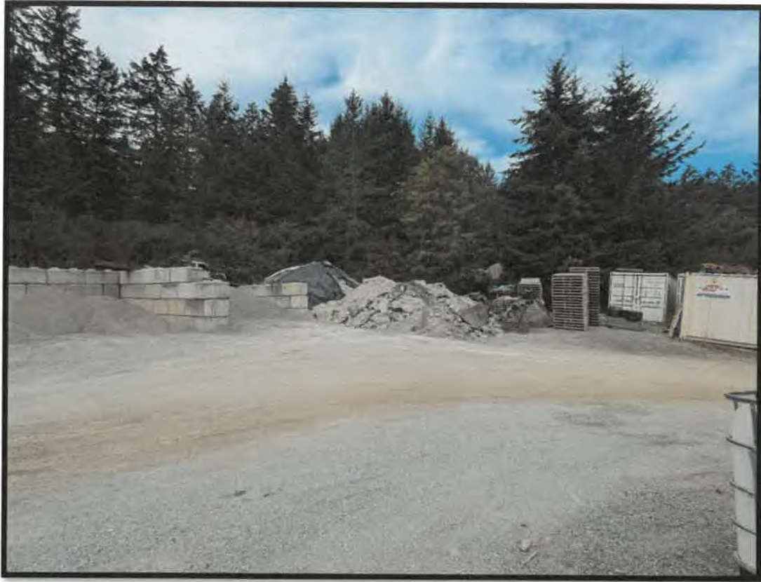
Photo 9: Stockpiled material to be covered prior to rainy season.
