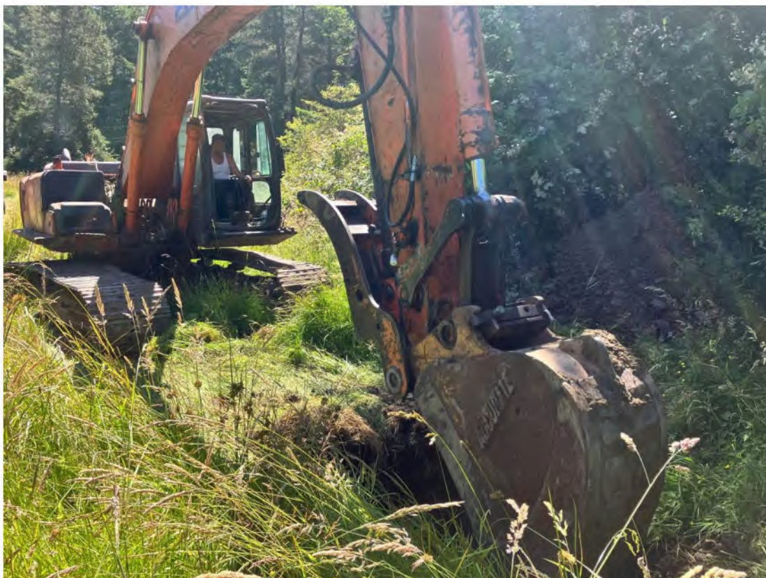
Photo 1. Excavator employed to install monitor well, June 30, 2025.
