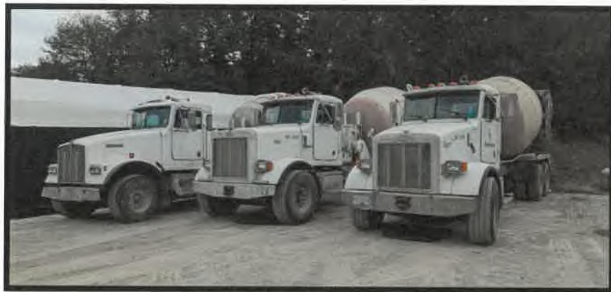
Photo 17: Drip trays noted below concrete trucks.
