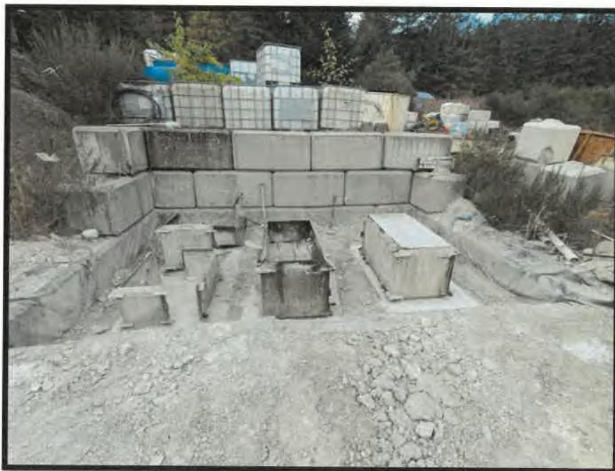
Photo 4: Lock block production area
