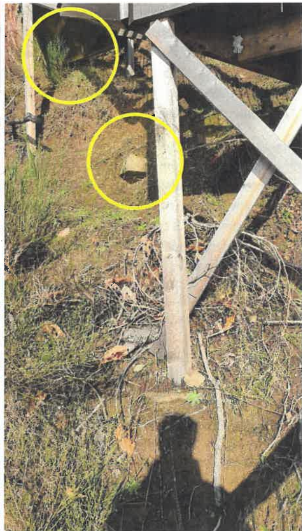
Photo 3 (below): Shows old, compromised footings (circled) in relation to current deck location.
