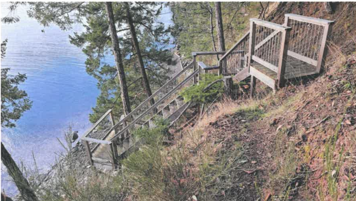
Photo 6: Looking down from the top of the slope - shows more stable soils with established Scotch broom and grass dominated understory.
