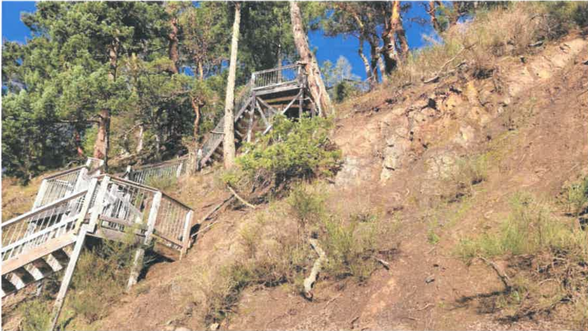
Photo 5: Looking up from the beach – shows area of erosion and exposed bedrock on right in relation to stairs on left. Note sparse vegetation established on erosion area indicating some stability, at least in the short-term.
