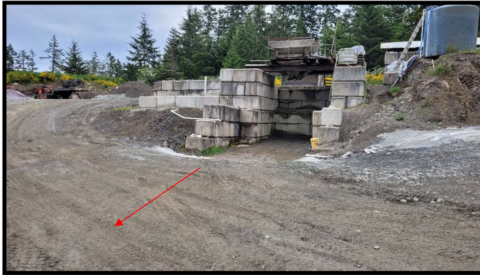
Photo 7 – Site grading improvements convey surface waters away from batching area.
