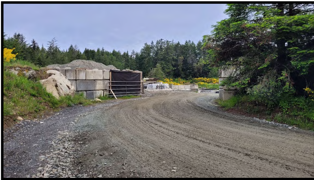
Photo 4 – Lockable gate at site entrance.
