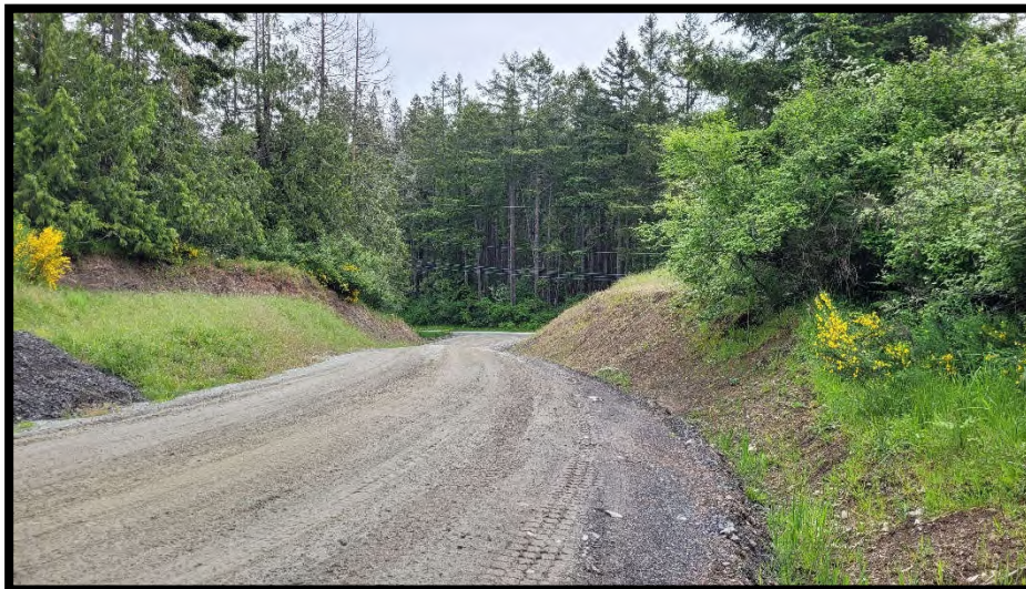
Photo 2 – Site Access ‘A’, complete with roadside ditching, gravel surfacing and stabilized banks.
