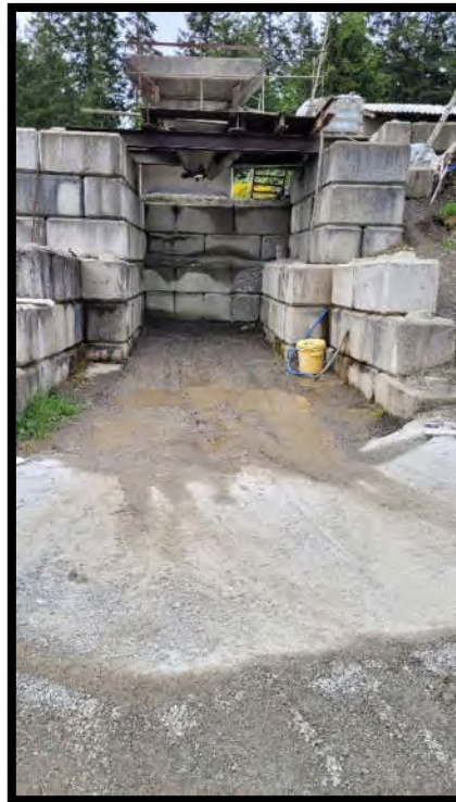
Photo 6 – Concrete batching area with enlarged concrete apron.
