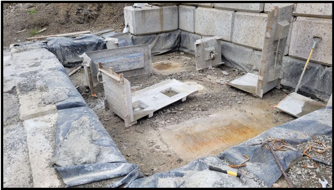
Photo 8 – Poly lined lock block fabrication cell.
