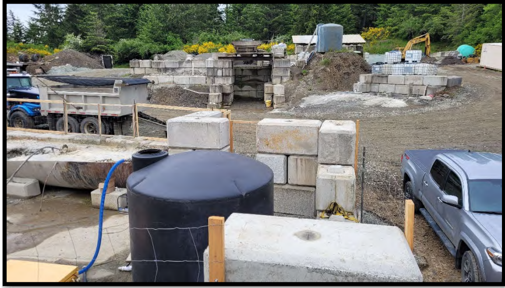
Photo 5 – Overview of site, looking south towards batching area.
