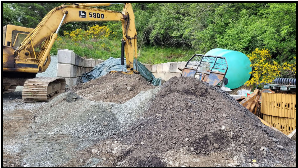
Photo 14 – Covered stockpile of waste concrete and mixed aggregate for reuse.
