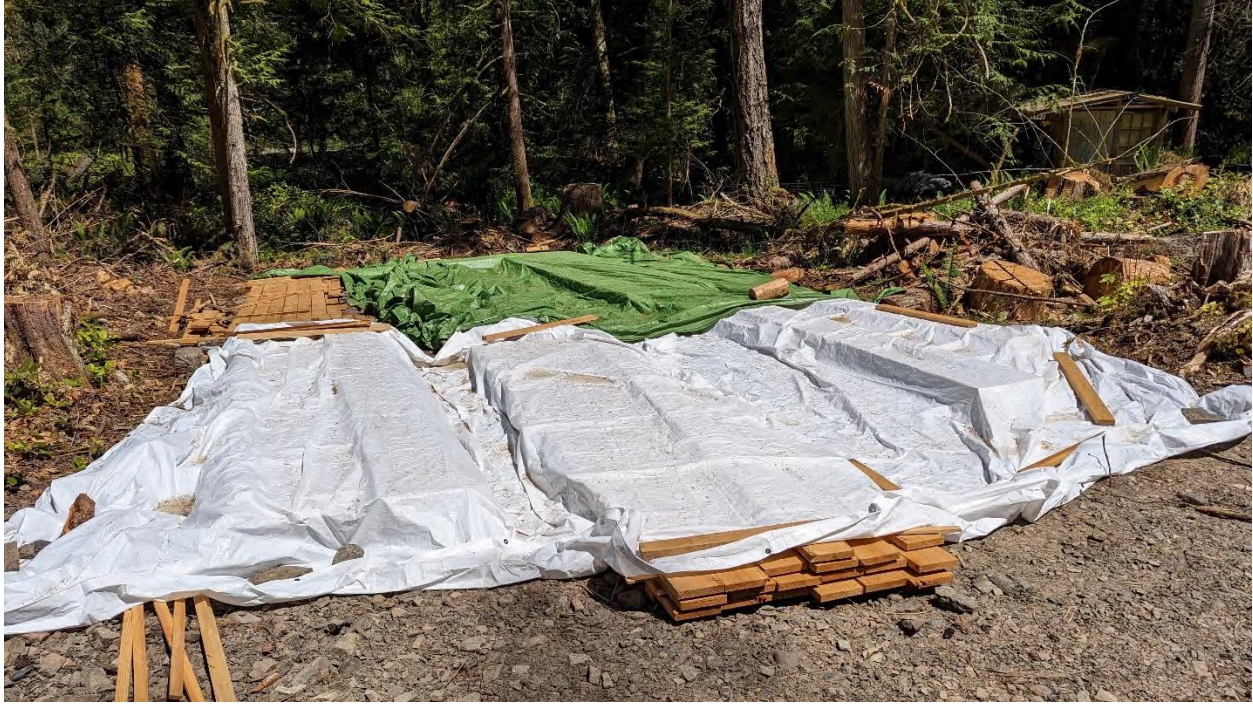
Photo 13 shows the cleared landing used for temporary storage of milled timber. The landing fronts on the newly added driveway/road.
