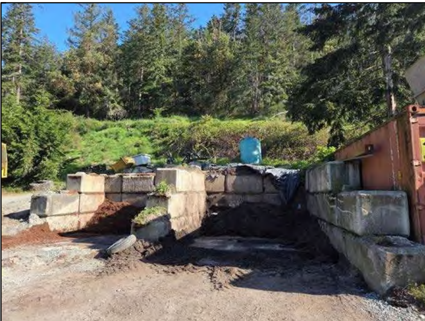
Photo 3: Soils are contained in lock block bins.
