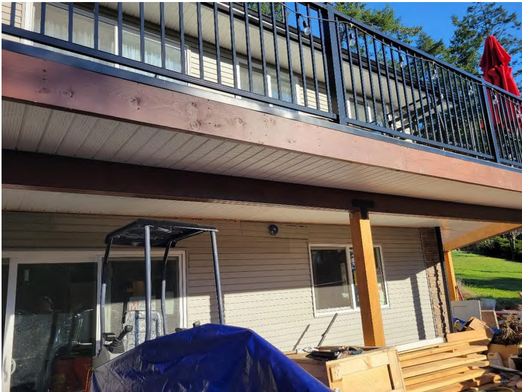
SOUTH-EAST CORNER OF SUITE LOOKING NORTH
