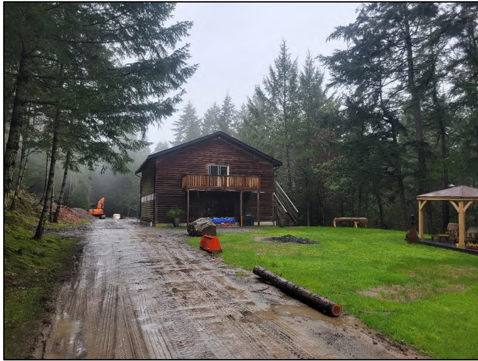
EXISTING BARN, LOOKING NORTH-WEST
