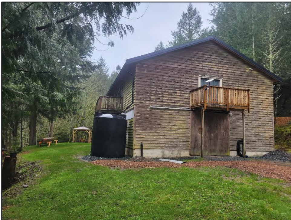
EXISTING BARN, LOOKING SOUTH-EAST
