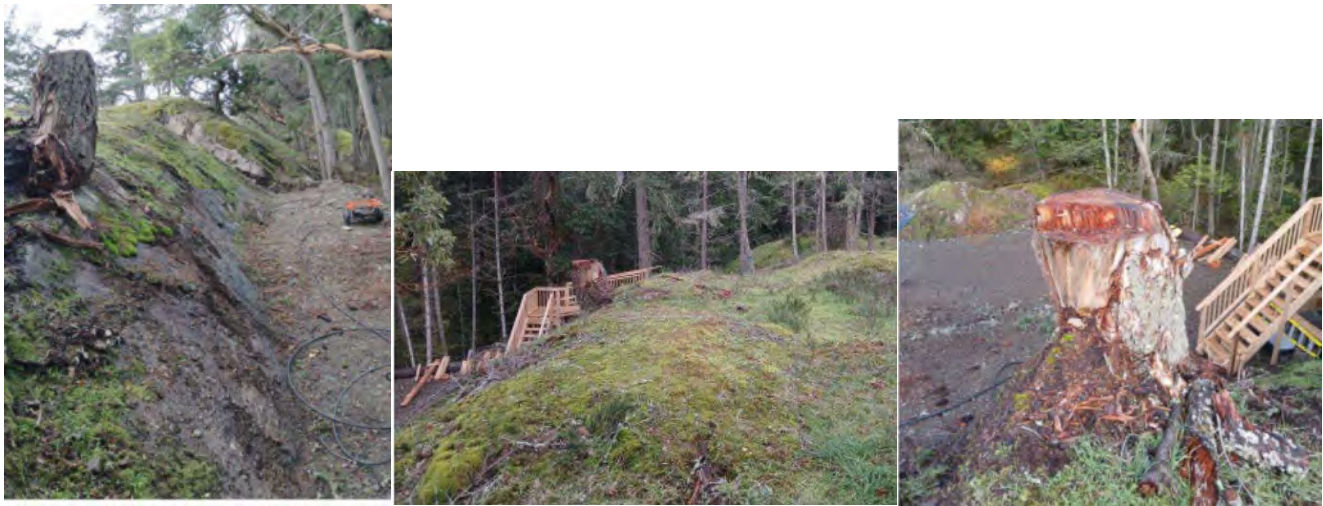
Figure 2. Unauthorized Tree Removal, Stair Construction and Land Clearing in DPA 2
