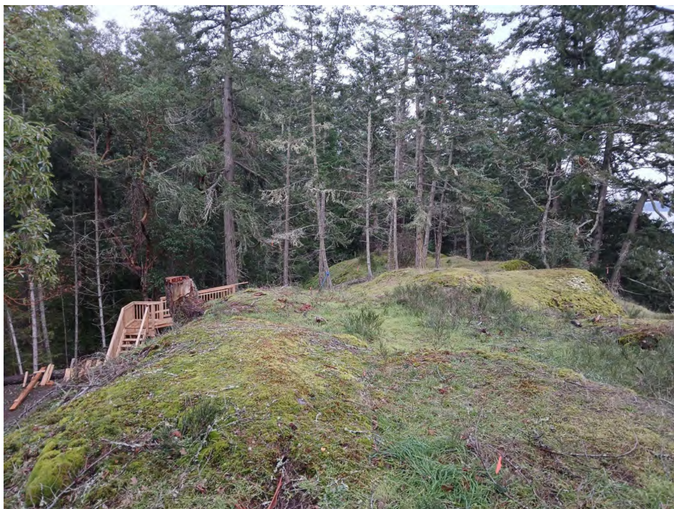
Plate 1. Newly constructed stairway against the bedrock surface in the Herbaceous Ecosystem DPA at 6915 Pirates Road, Pender Island, BC. Felled veteran Douglas-fir stump also visible in front of stairs.
