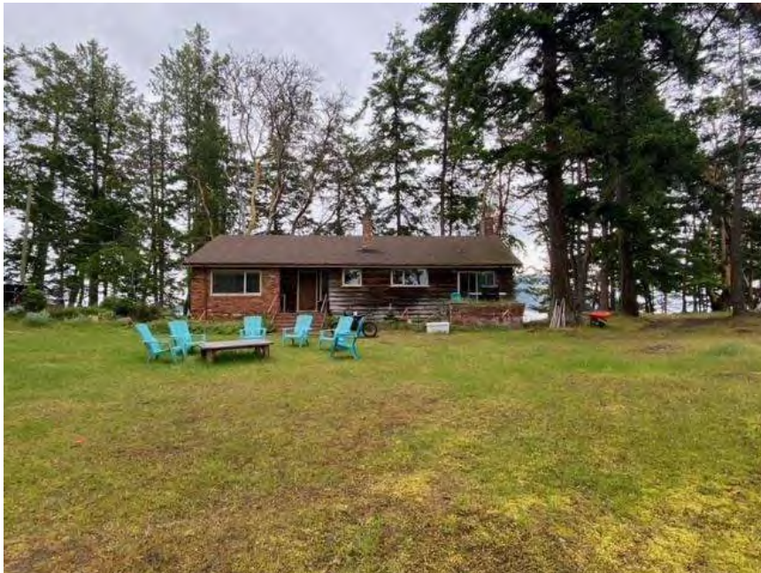
PHOTO 2. - HOUSE TO BE REMOVED - NORTHERN PERSPECTIVE
