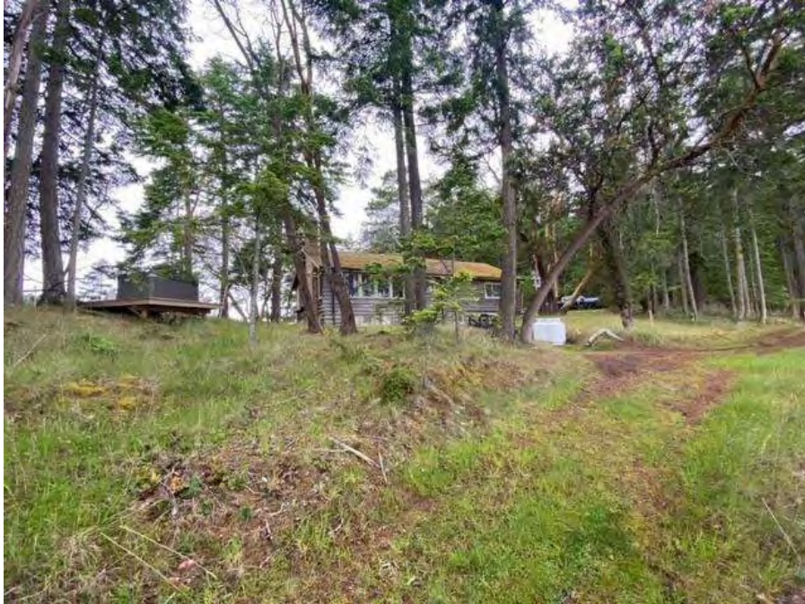
PHOTO 5. - HOUSE TO BE REMOVED – REARVIEW
