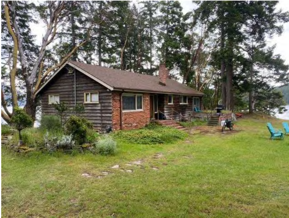
PHOTO 1. HOUSE TO BE REMOVED – NORTHWESTERN PERSPECTIVE
