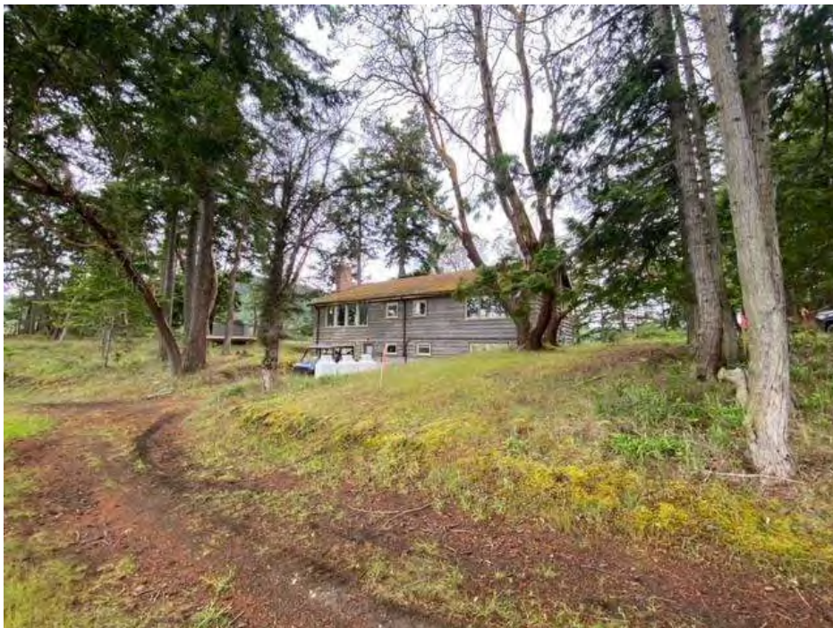
PHOTO 6. - HOUSE TO BE REMOVED – AREA FOR NEW HOUSE TO BE LOCATED
