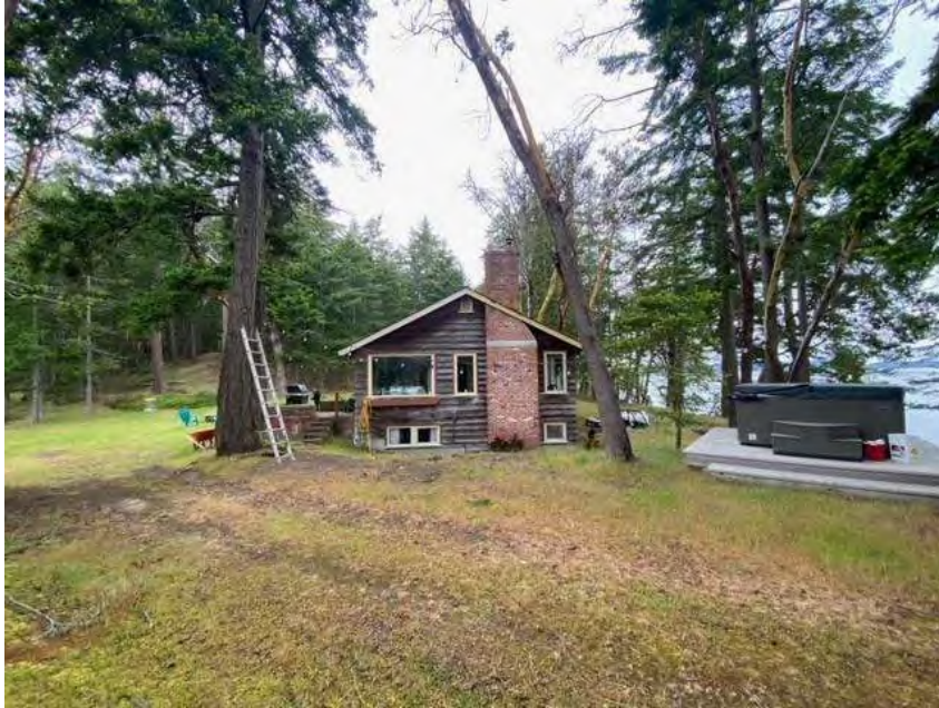
PHOTO 3. - HOUSE TO BE REMOVED – VIEW FROM EASTERN PERSPECTIVE
