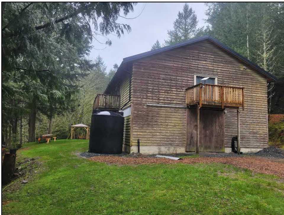
EXISTING BARN, LOOKING SOUTH-EAST
