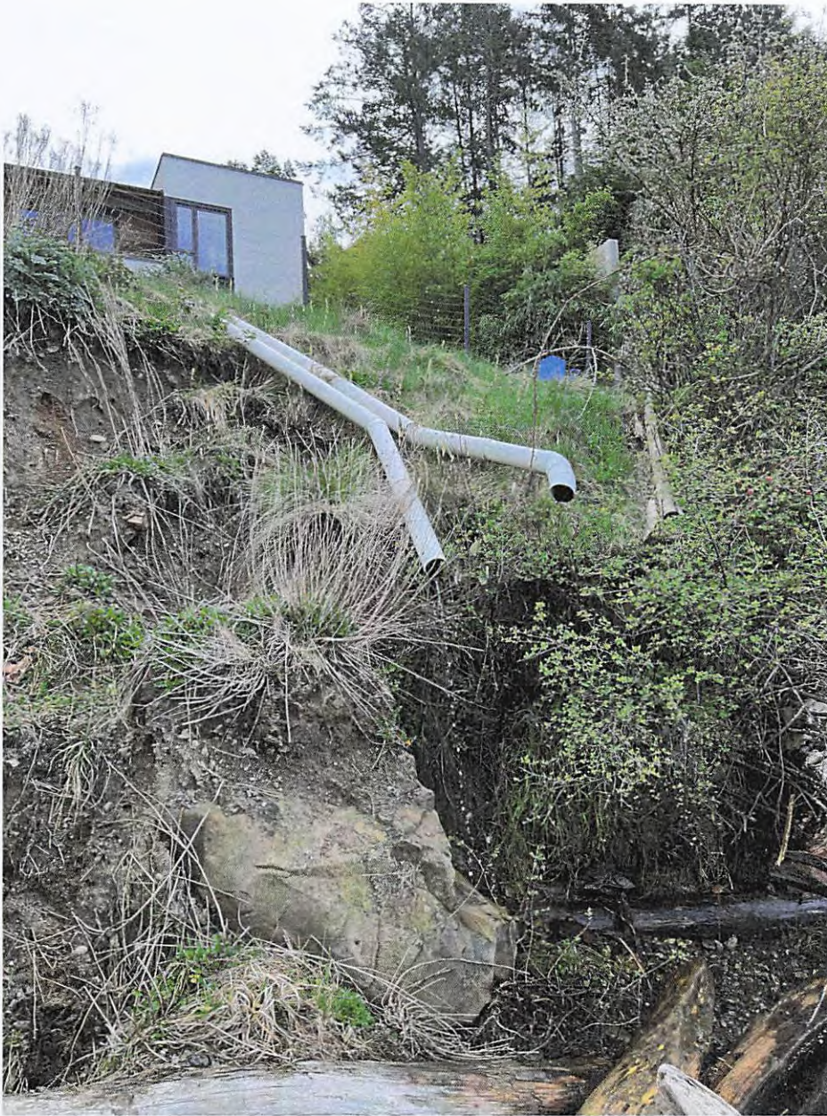
Photo 2. Twinned perforated drainage pipes south of stairs.
