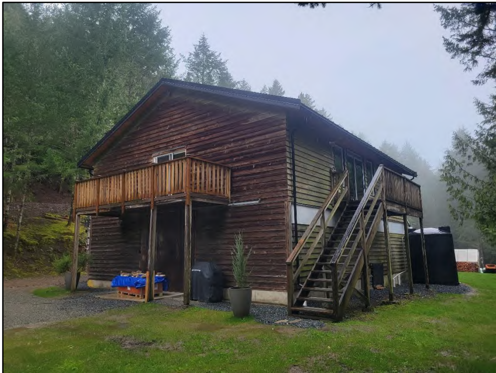
EXISTING BARN, LOOKING WEST
