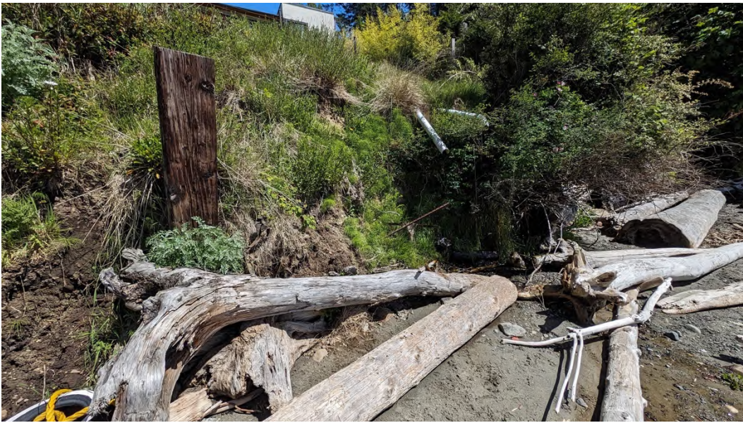
Photo 3. Looking south along the beach at the shoreline and base of eroding slope (May 2024). Additional soil slippage has occurred in winter 2024/2025 – see Photos 10-12.
