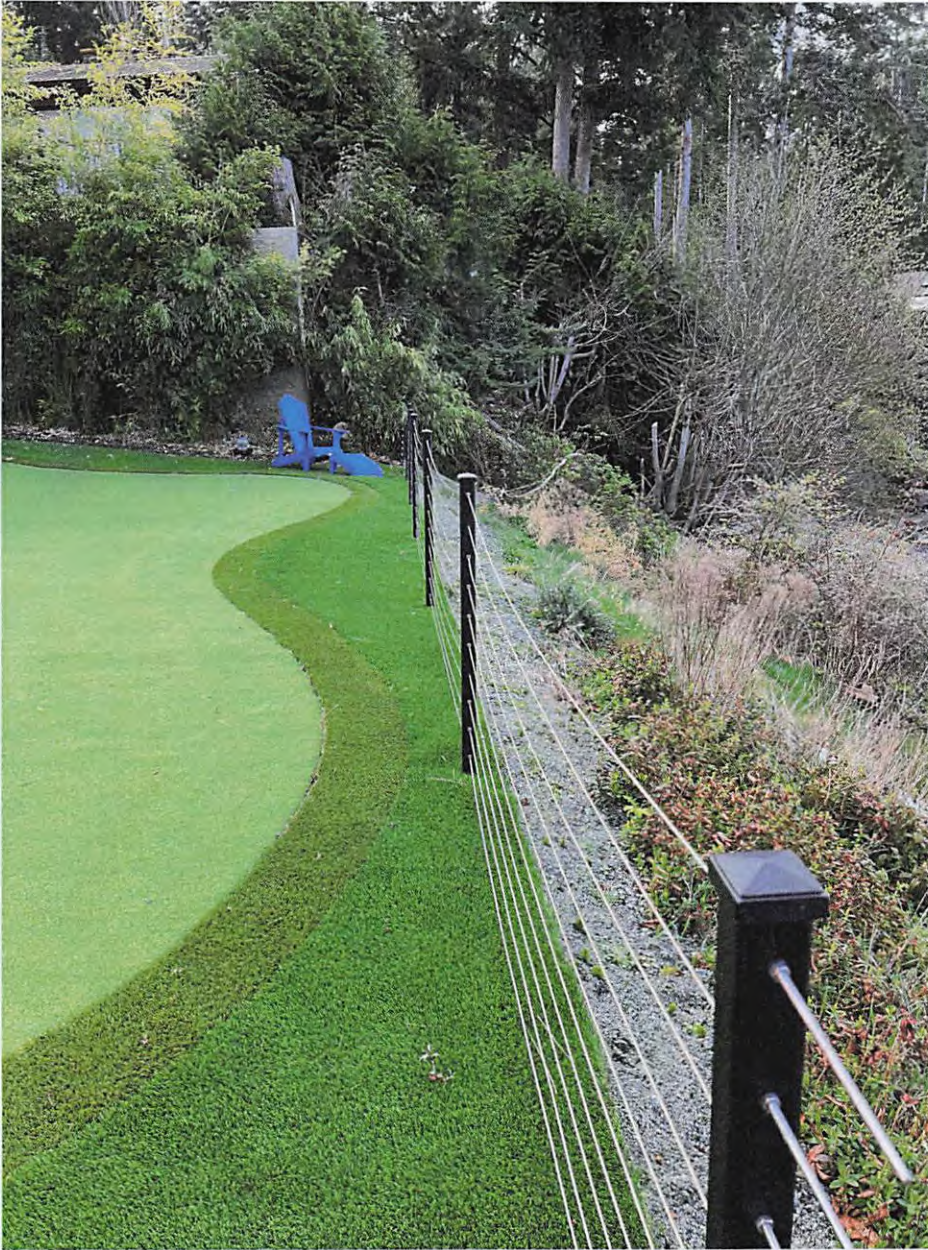
Photo 5. Looking south along crest of slope. Curvature at crest visible in distance.
