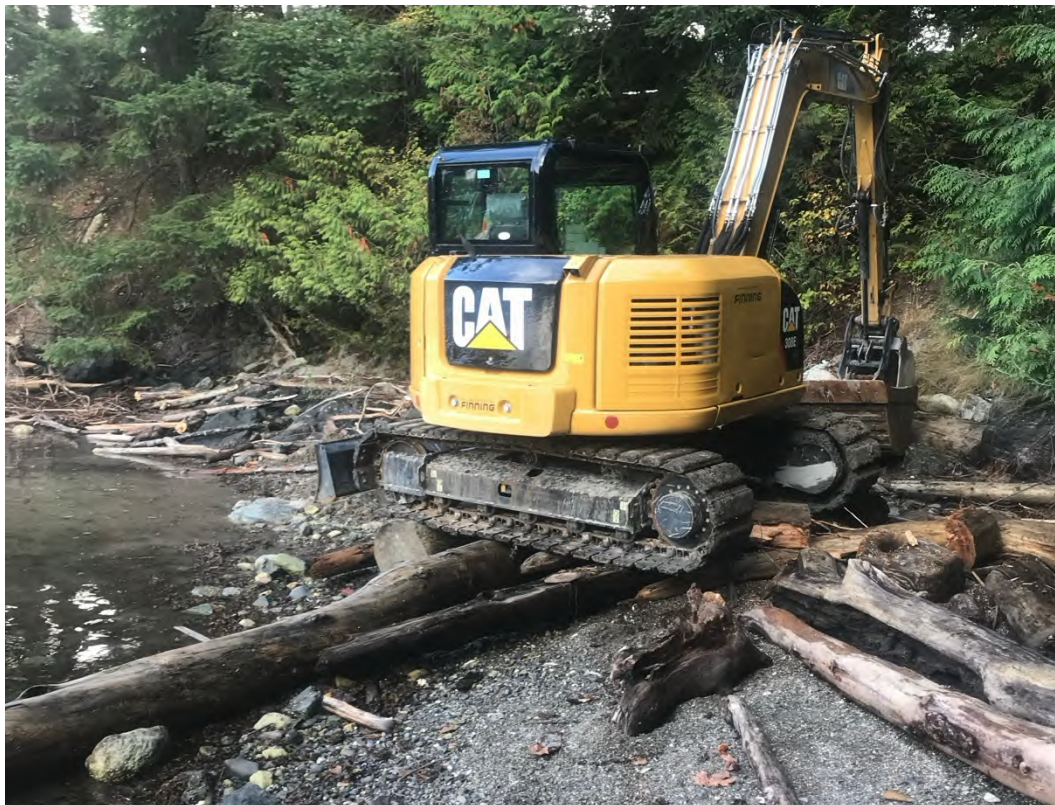
Photo 17. Excavator to be stored above wave action, if needed, on bunked logs, with floating spill boom around.
