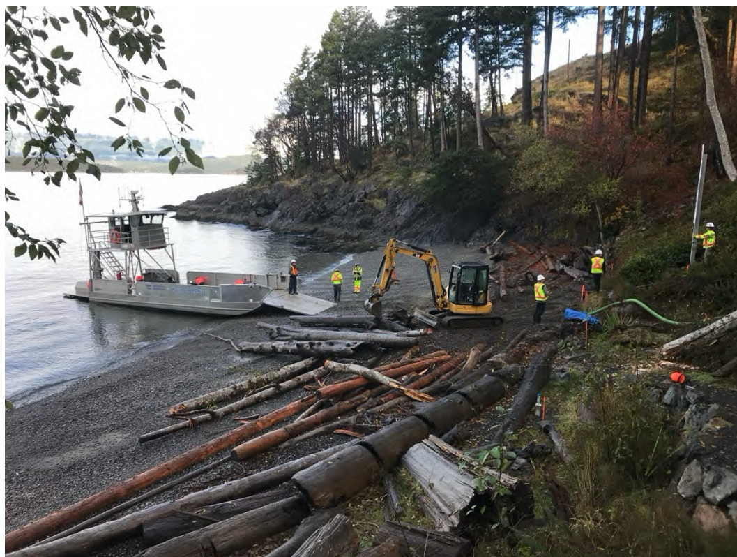
Photo 18. Small self-propelled barge with ramp for bringing equipment and materials to the site.
