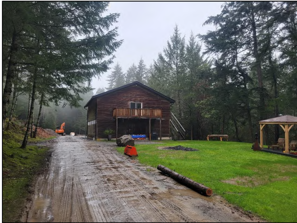
EXISTING BARN, LOOKING NORTH-WEST
