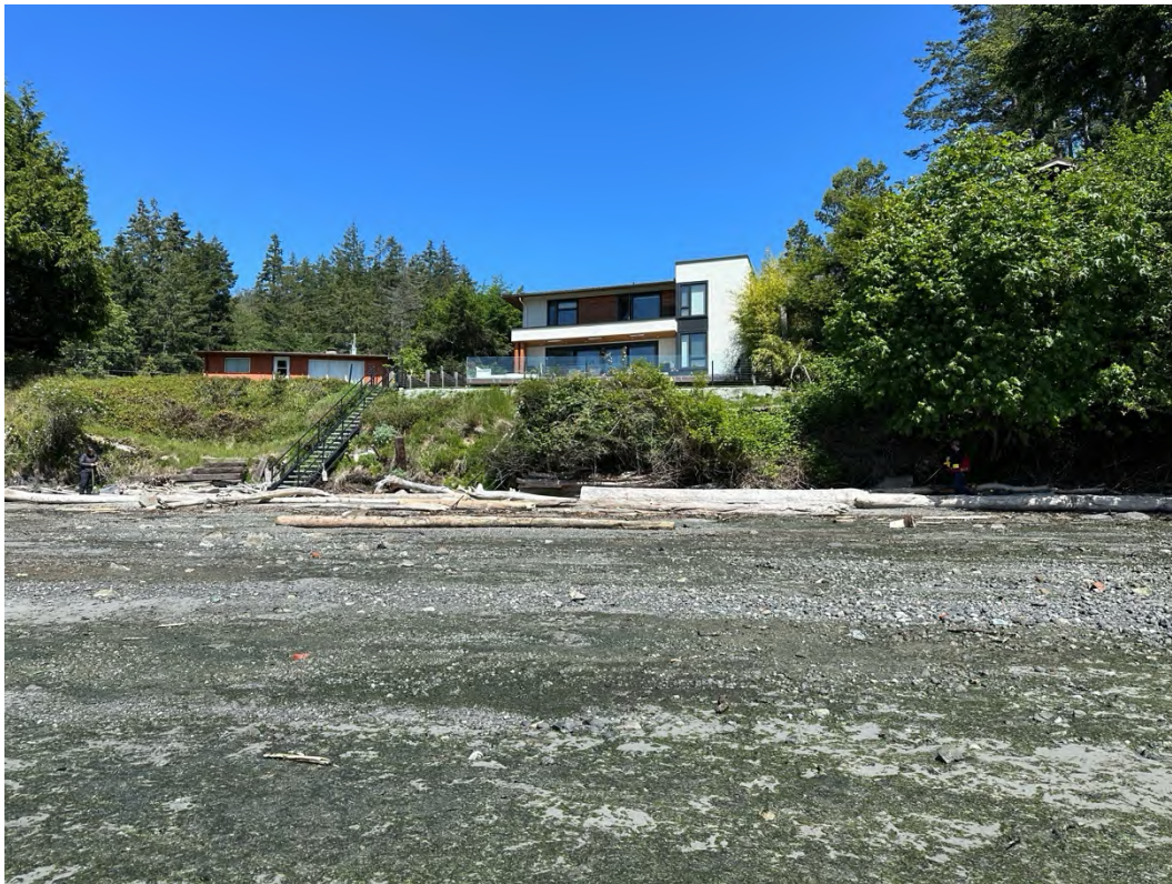
Photo 13. Beach access to the site for barge landing and equipment access.
