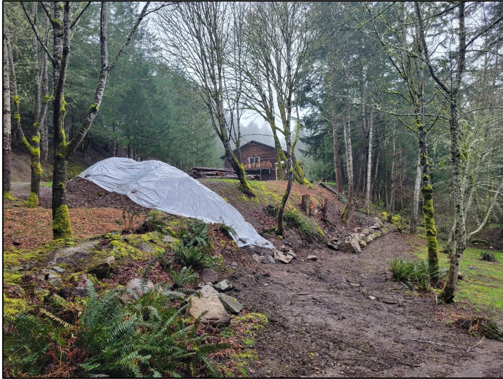
EXISTING BARN, VIEW FROM DRIVEWAY LOOKING NORTH-WEST
