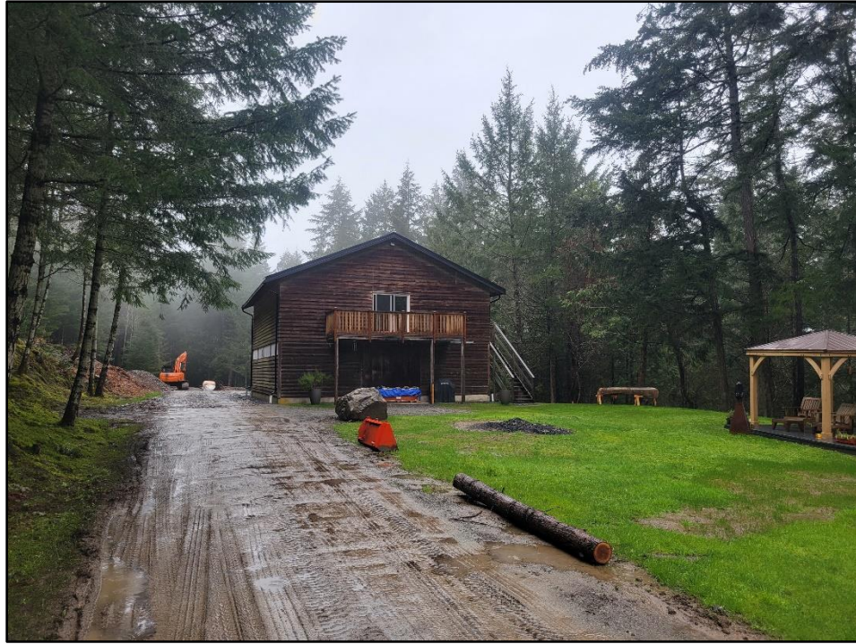
EXISTING BARN, LOOKING NORTH-WEST
