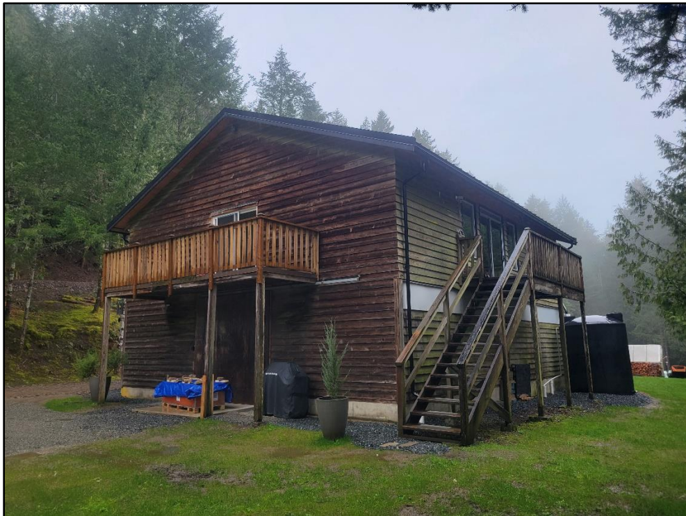
EXISTING BARN, LOOKING WEST
