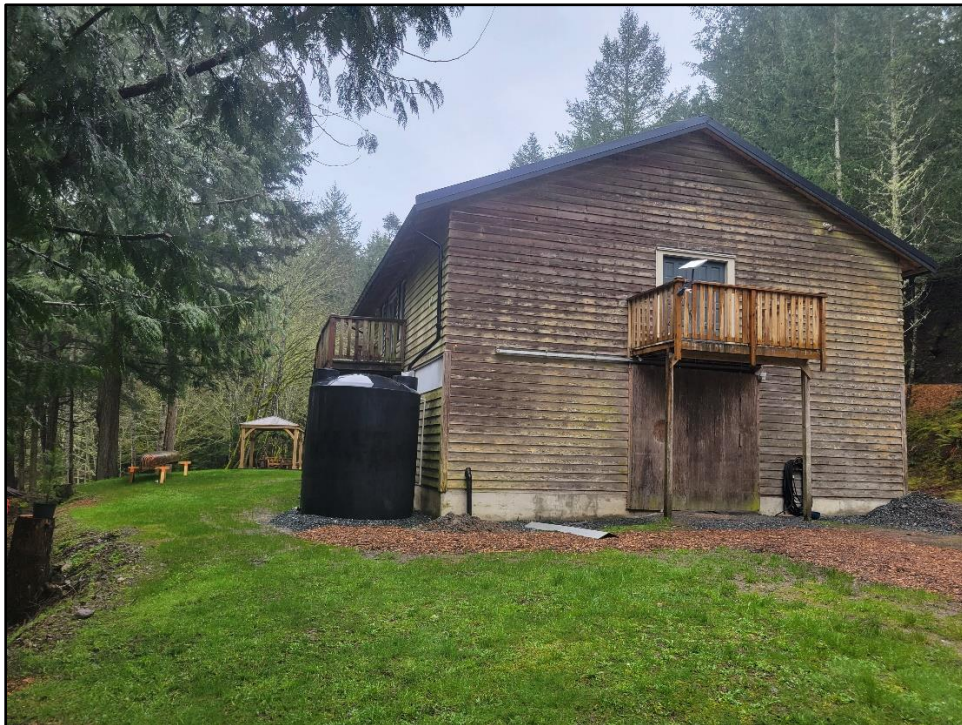
EXISTING BARN, LOOKING SOUTH-EAST
