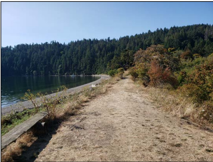
Photo 7. Looking south along the top of the shoreline berm.
