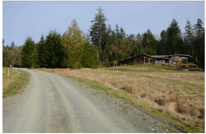
Driveway and Single-Family Dwelling on Subject Property
