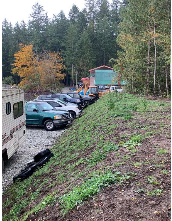
Photo 4: Berming of soil on Southern boundary of parking area.
