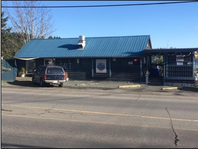
Image 1 – Existing building on subject property.
