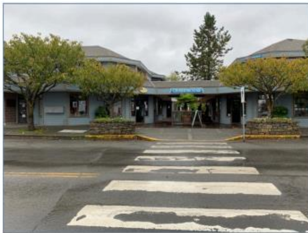
6. Connection from Fulford Ganges Road
