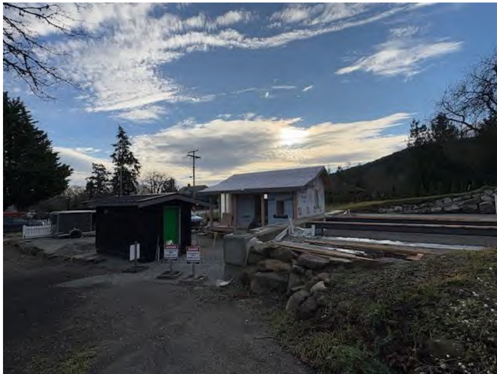
Figure 6 – Electrical Shed & Concrete Blocks
