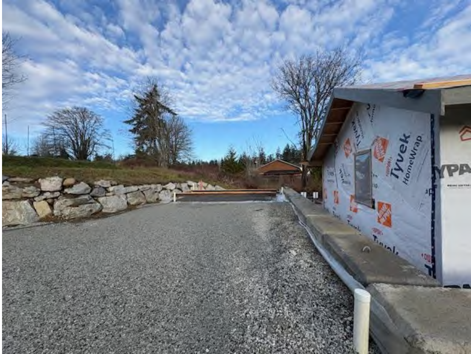
Figure 8 – Concrete Blocks, Building B and the proposed location for building A
