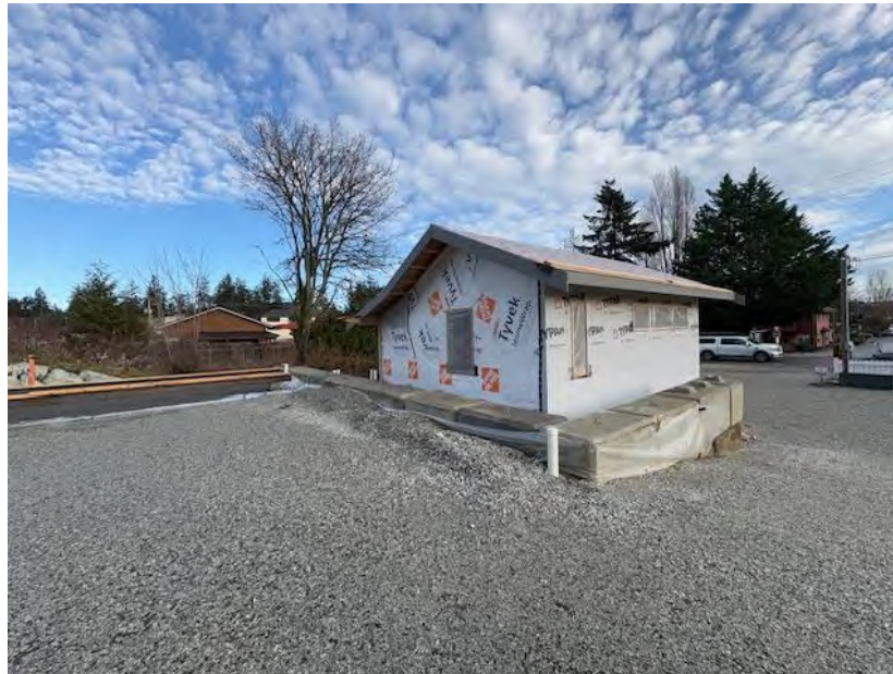
Figure 11 – Concrete Blocks, Building B and the proposed location for building A
