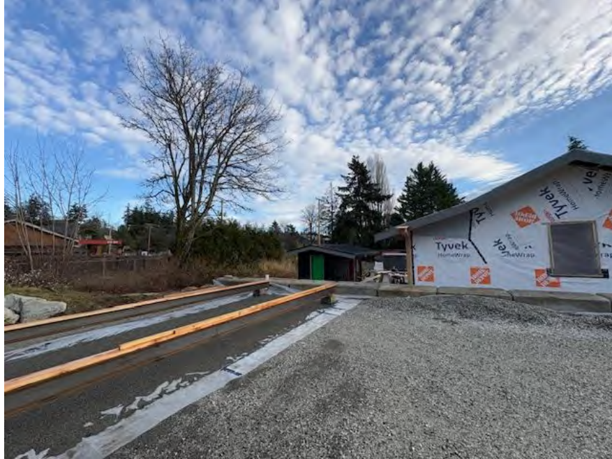
Figure 8 – Concrete Blocks, Building B, proposed location for building A and Electrical Shed
