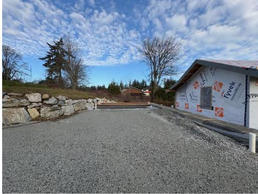
Figure 10 – Concrete Blocks, Building B and the proposed location for building A (South view)
