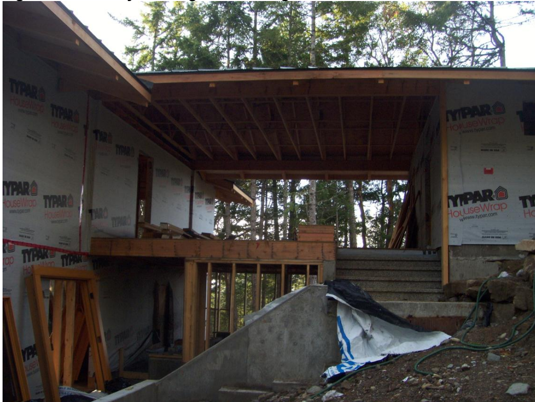
Figure 2 Accessory Building and Dwelling
