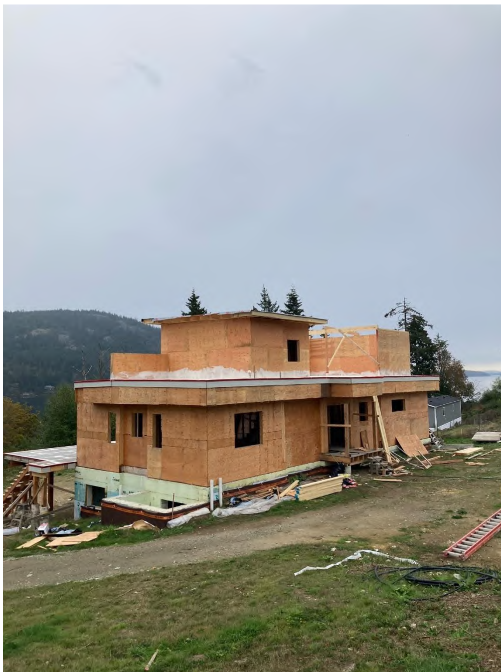
Figure 12 - View from Isabella Point Road
