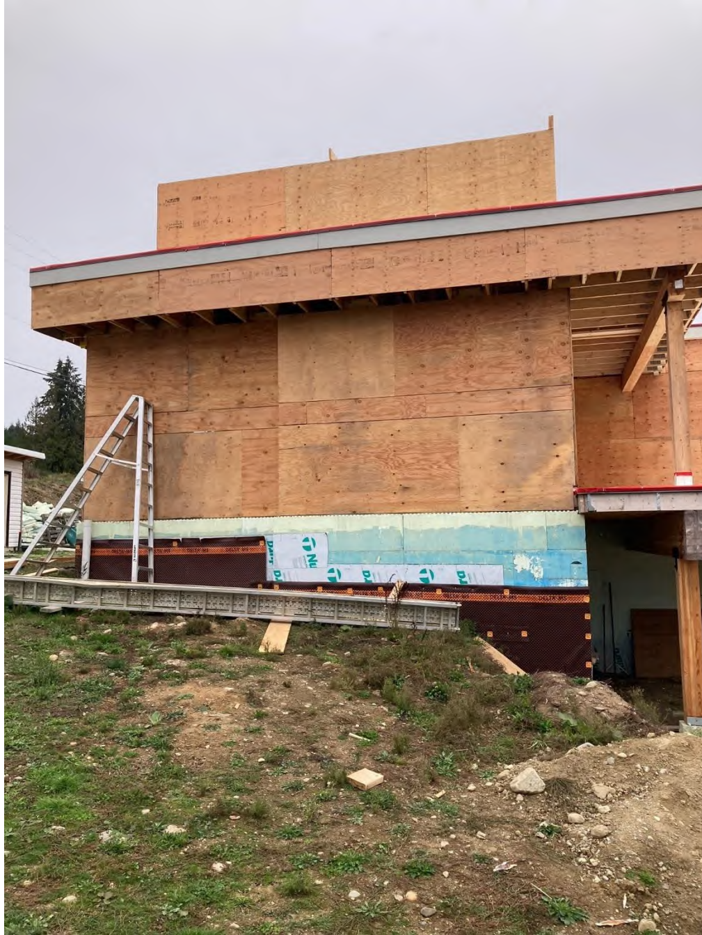
Figure 14 - South East Elevation 2
