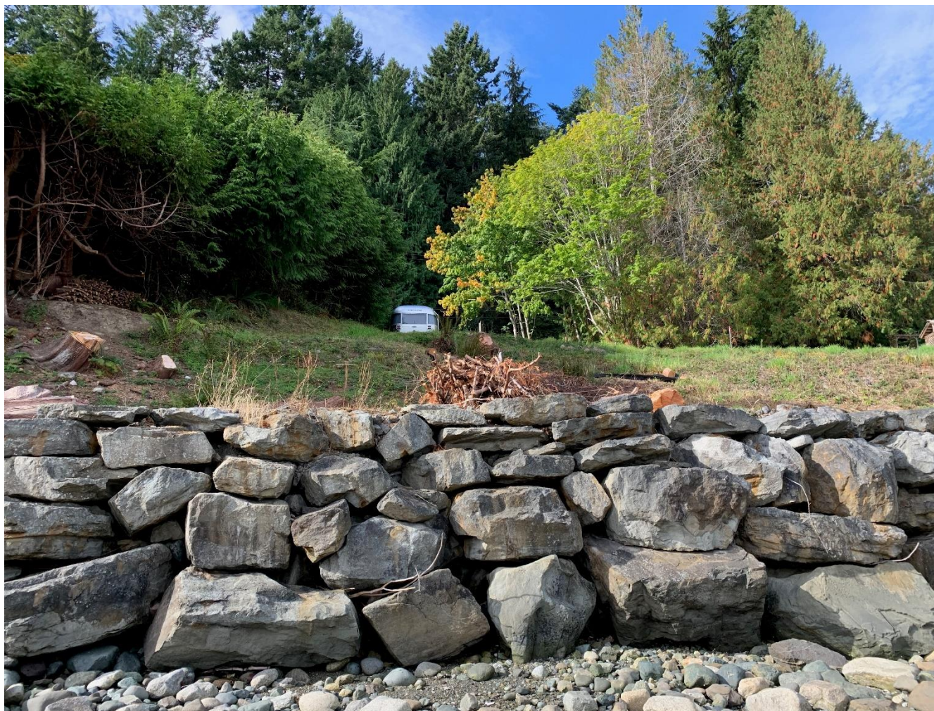
PHOTO 4: RETAINING WALL LOOKING WEST FROM BEACH
