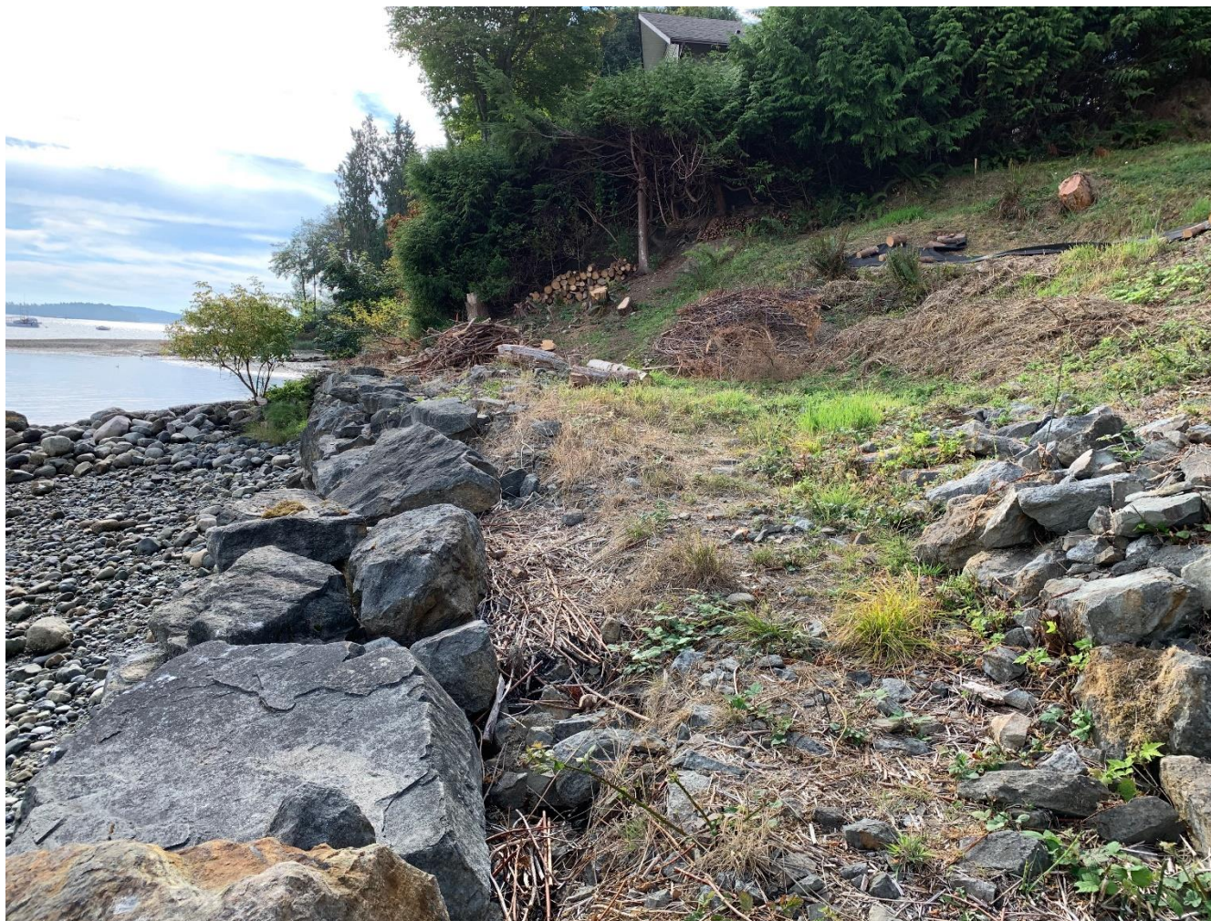
PHOTO 5: RETAINING WALL LOOKING SOUTH
