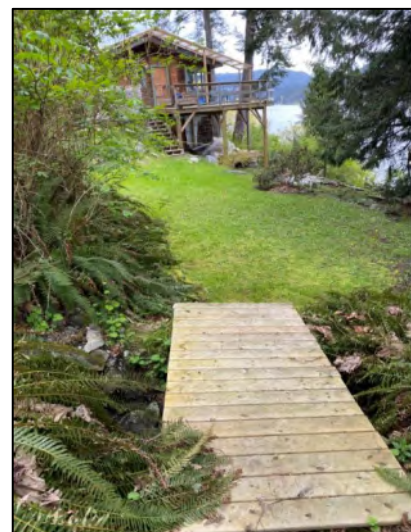
Figure 6 Existing bridge over watercourse at front of property
