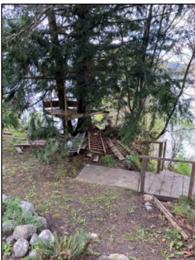
Figure 5 Existing treehouse with building materials
