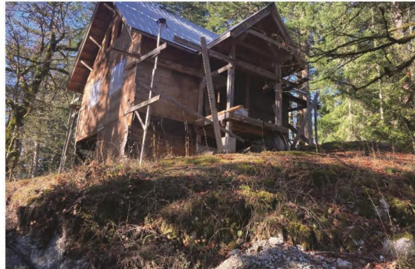
Seasonal Cottage Under Construction (North of Beaver Point Road)
